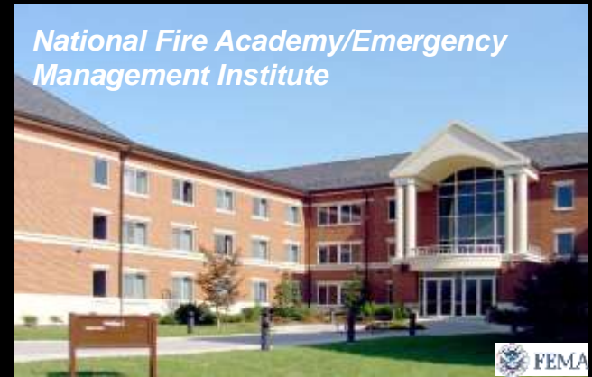
Community-Specific Integrated Emergency Management Course (CS IEMC) - Earthquake Hazard - April 14 – 18, 2014 Emmitsburg, MD
