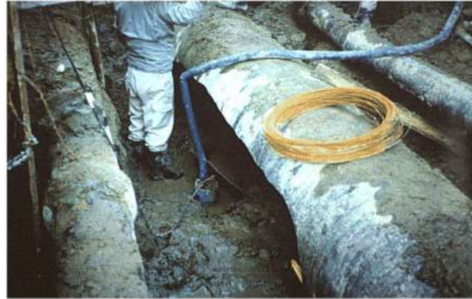
Burst cast iron pipe. Kobe 1995
