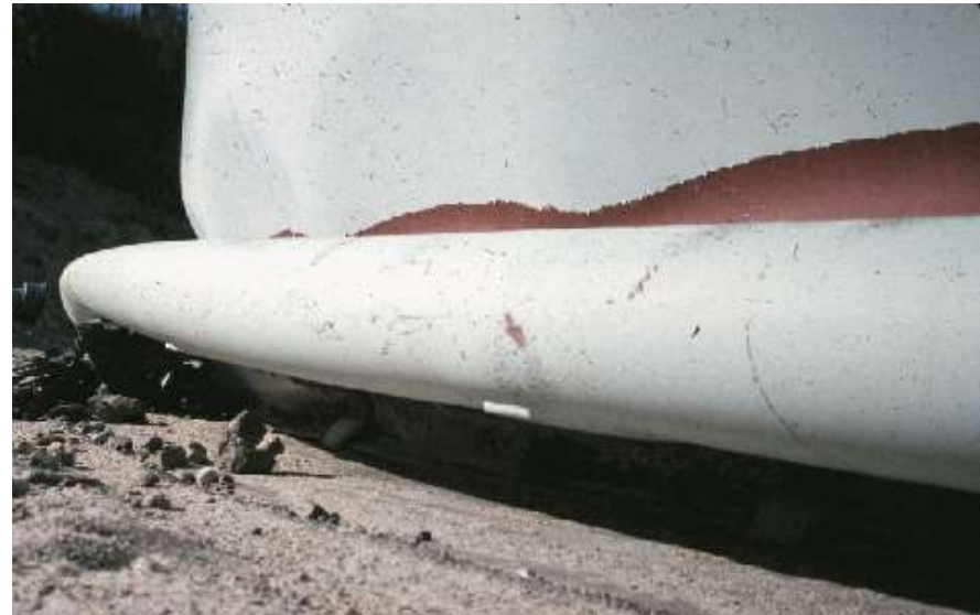
Buckled Steel Tank. Northridge Earthquake, 1994
