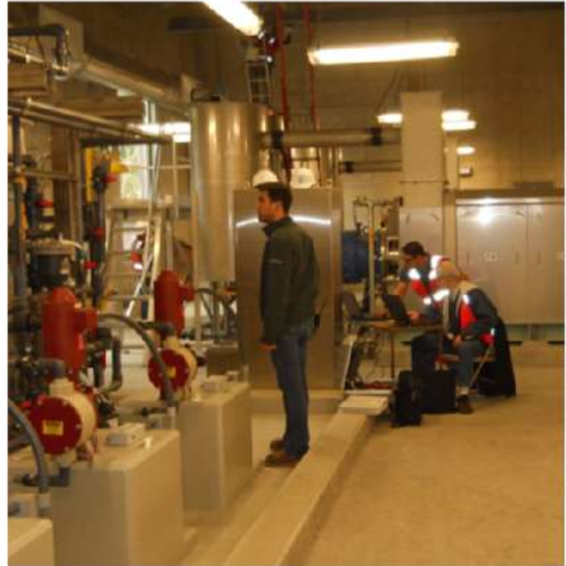
COMMISSIONING AND STARTUP
