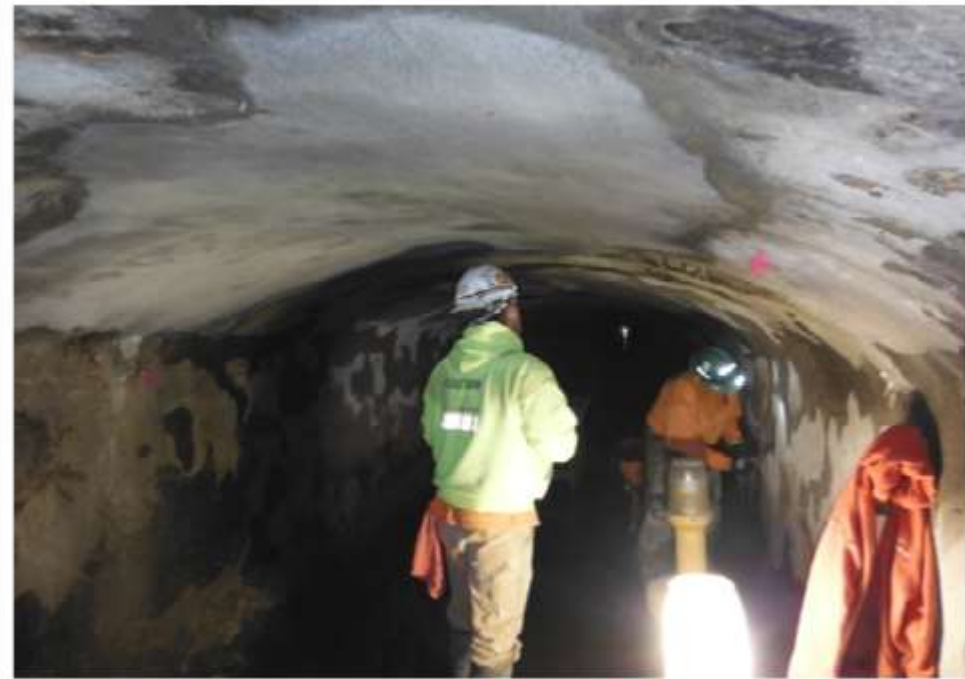
Tunnel After Repair Work
