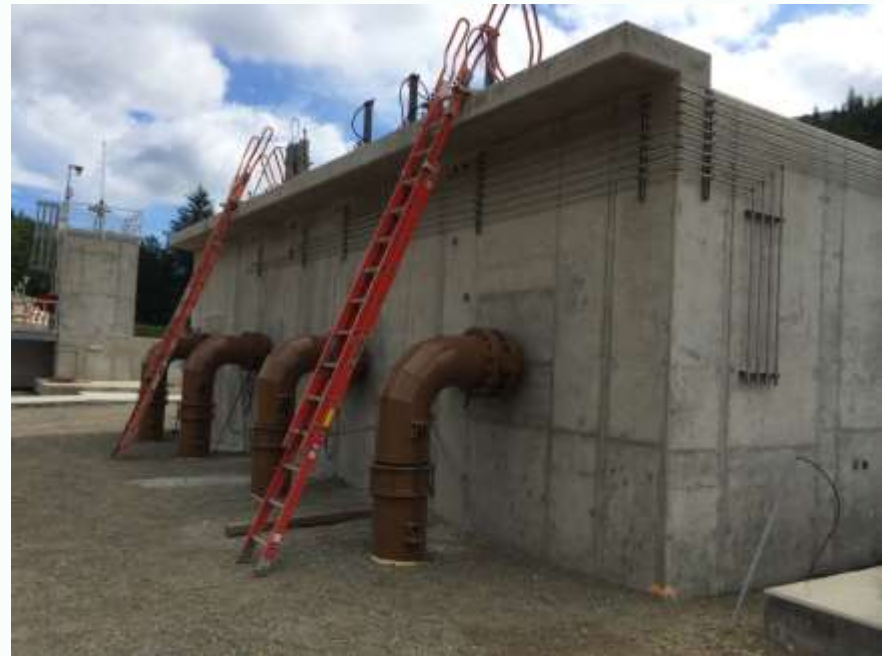
Inflow pipes from Washwater EQ Basins Pump Station
