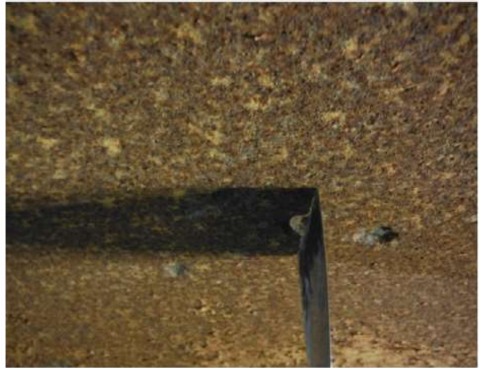
1930's Pipe Pitting Before Repair Work
