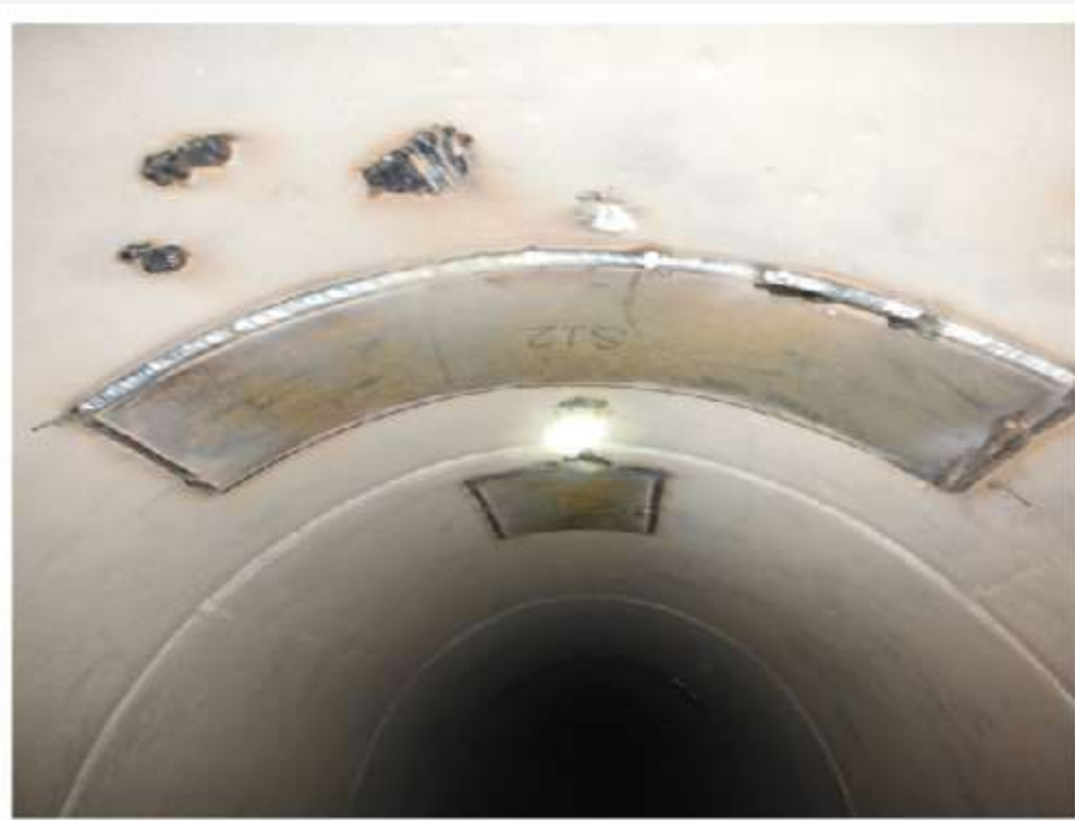
1930's Pipe During Repair Work (prior to polyurea lining)
