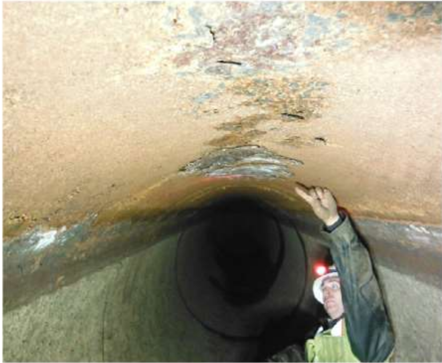
1930's Pipe Before Repair Work
