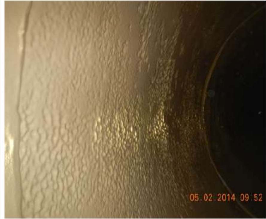
1930's Pipe After Repair Work
