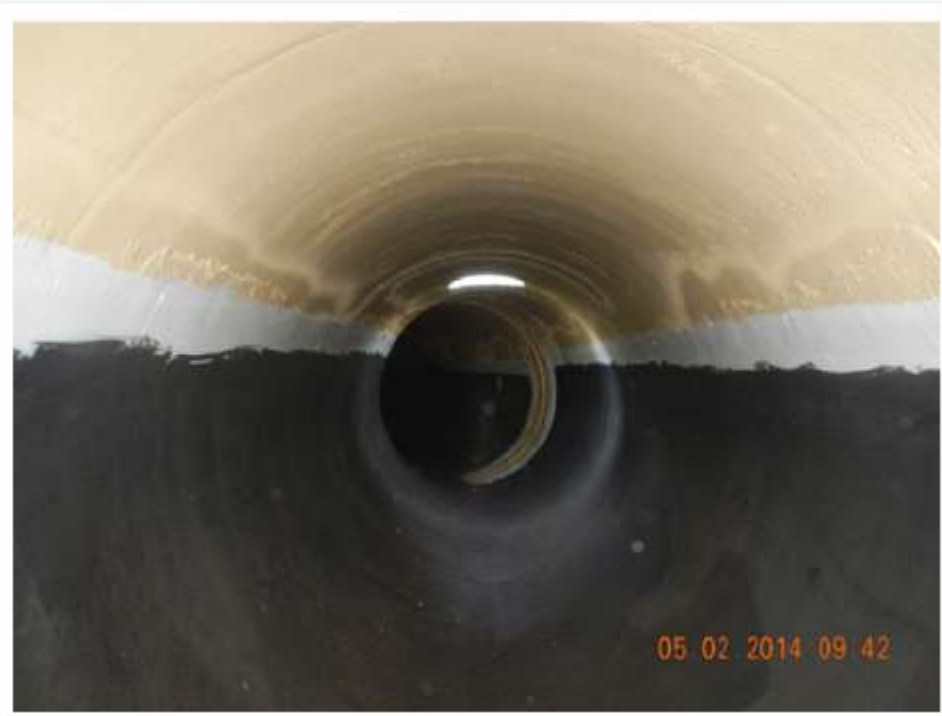
1960's Pipe After Repair Work
