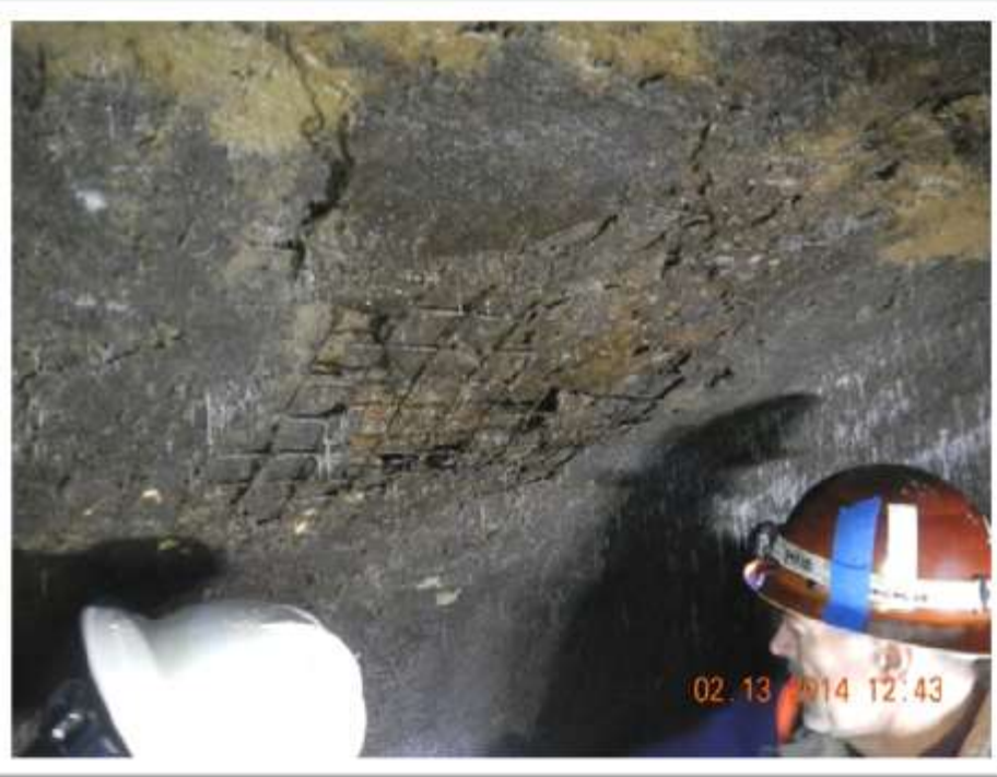
Tunnel Before Repair Work
