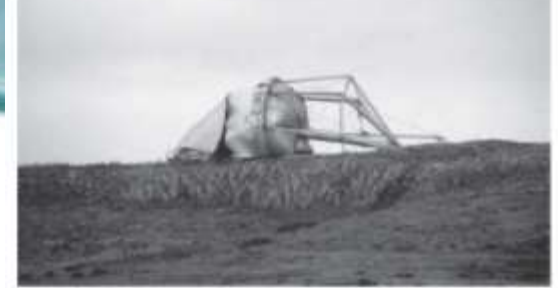
A water tower that has exceeded its useful life!
