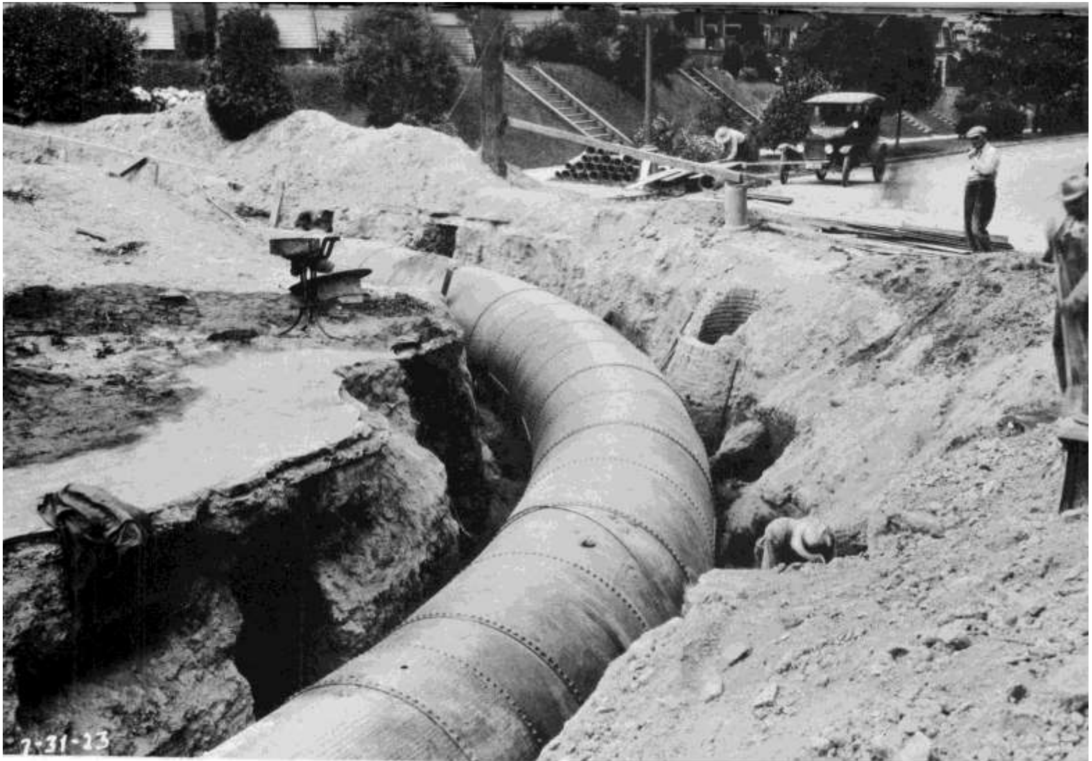
66" Steel Cedar River Pipeline at 18th Ave East & Prospect Street Under construction in 1923
