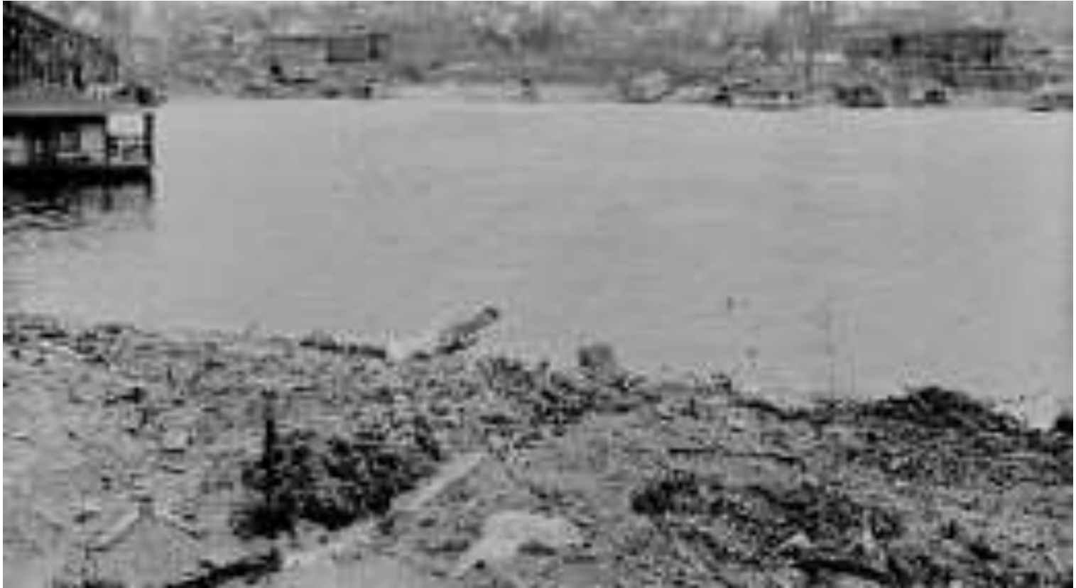
Lake Union sewer overflow
