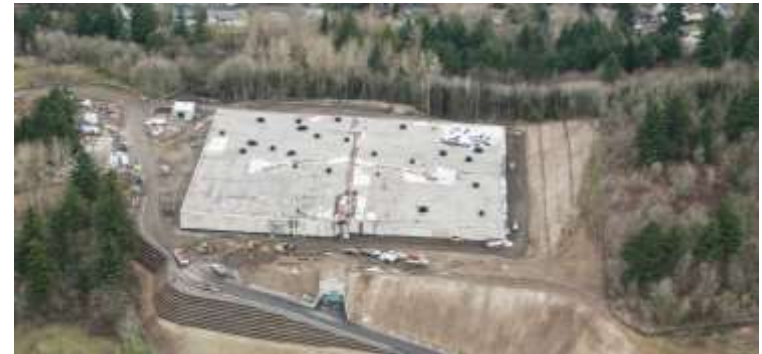
Buried Concrete Reservoir
