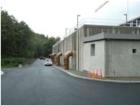
Above-Ground Process Basin at Water Treatment Plant
