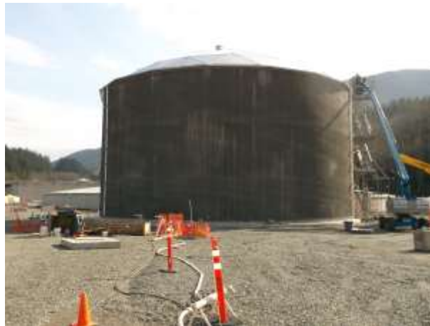
Circular Prestressed Concrete Water Tank
