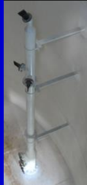
Passive TMS installed in tank
