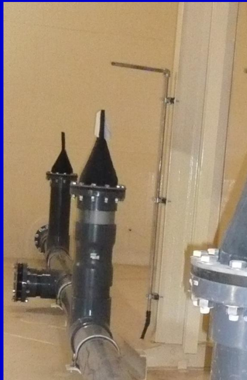
Into Tideflex Jet In Tank
