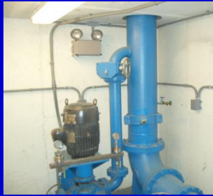
Passive TMS + Recirculation Pump (Mechanical Components Outside of Tank, Passive TMS Inside of Tank)
