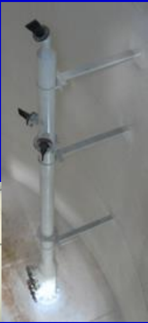
Passive TMS + Recirculation Pump (Mechanical Components Outside of Tank, Passive TMS Inside of Tank)
