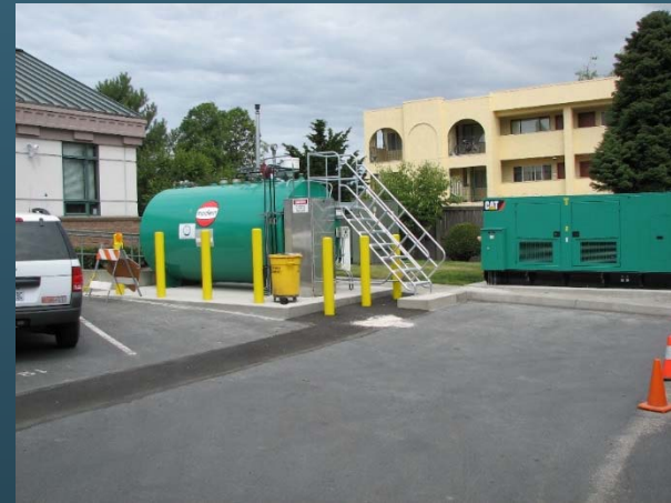
Replacement Generator and Fuel System
