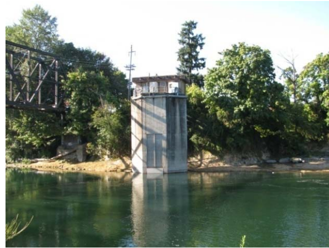
River Intake Pump Station (RIPS)
