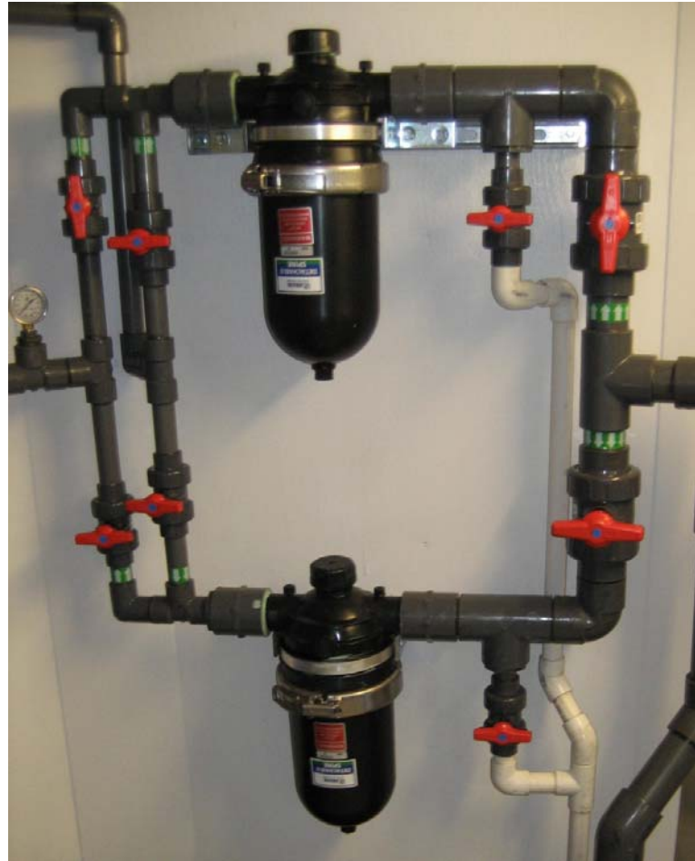
Ceramic Filters 20 micron
