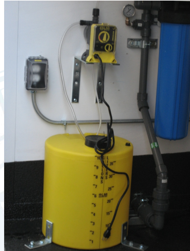
Chlorine Dosing Pump and Tank
