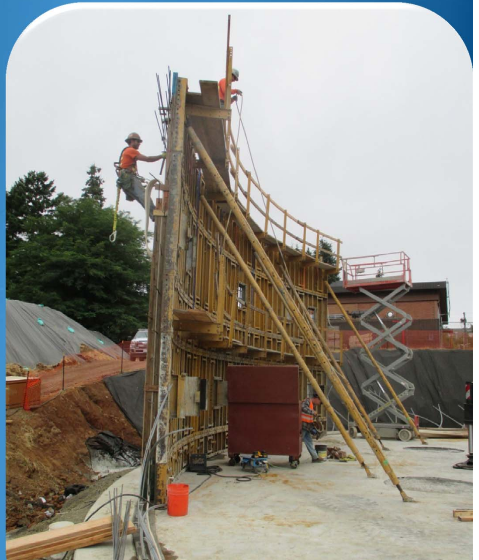
Multiple cast-in-place wall segments
