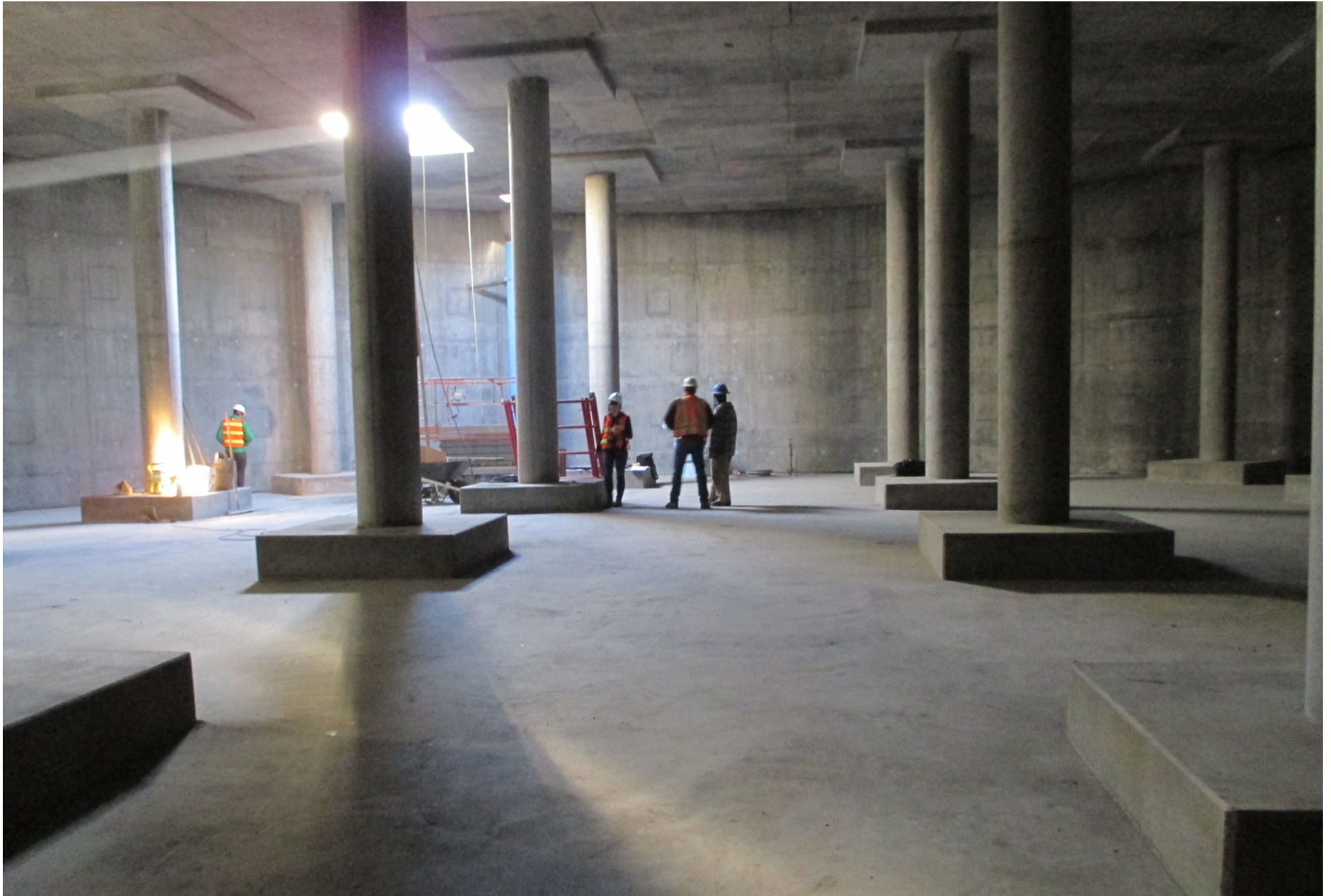
Reservoir Interior: Column-supported roof
