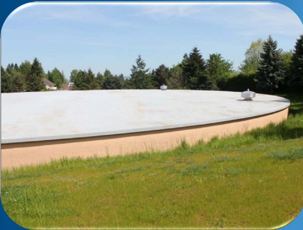
Concrete Reservoir, Tigard, OR
