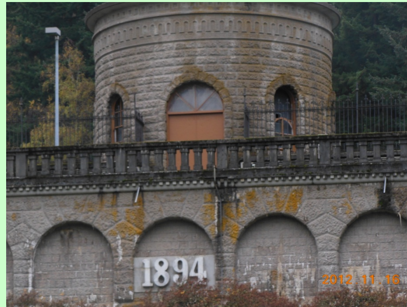
Washington Park Reservoir Improvements
