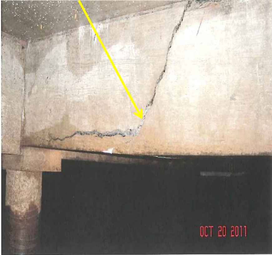
Photo 1: New beam failure east of south-central column
