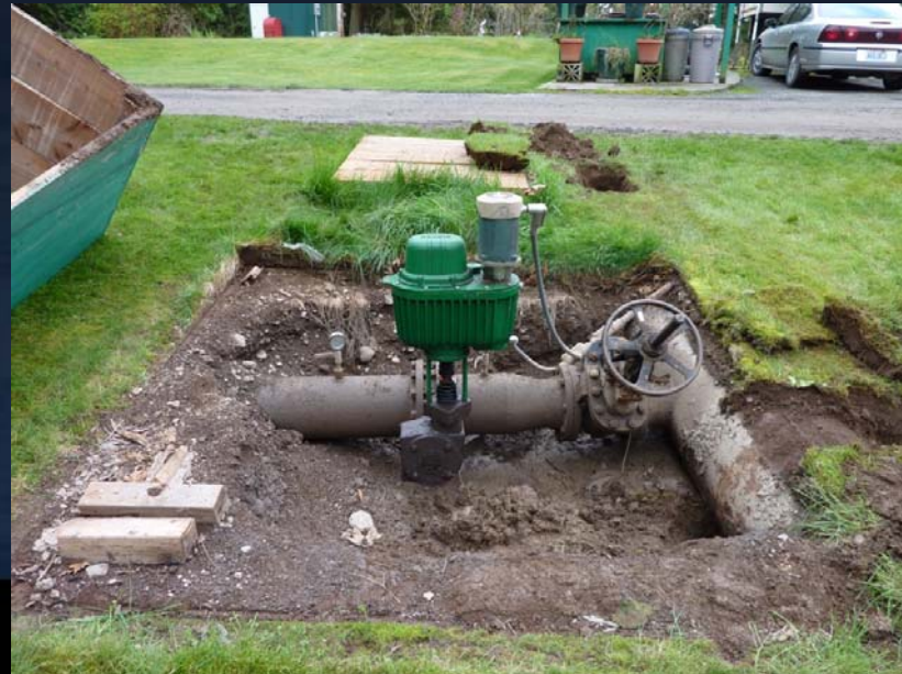
10-inch Isolation Valve (motorized)
