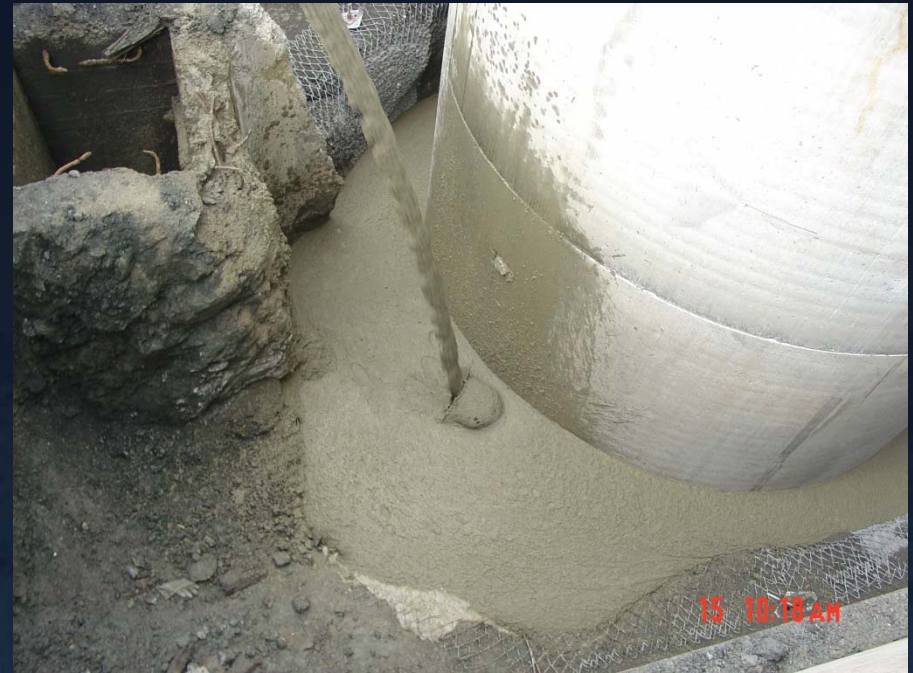
CDF backfill around the Shaft
