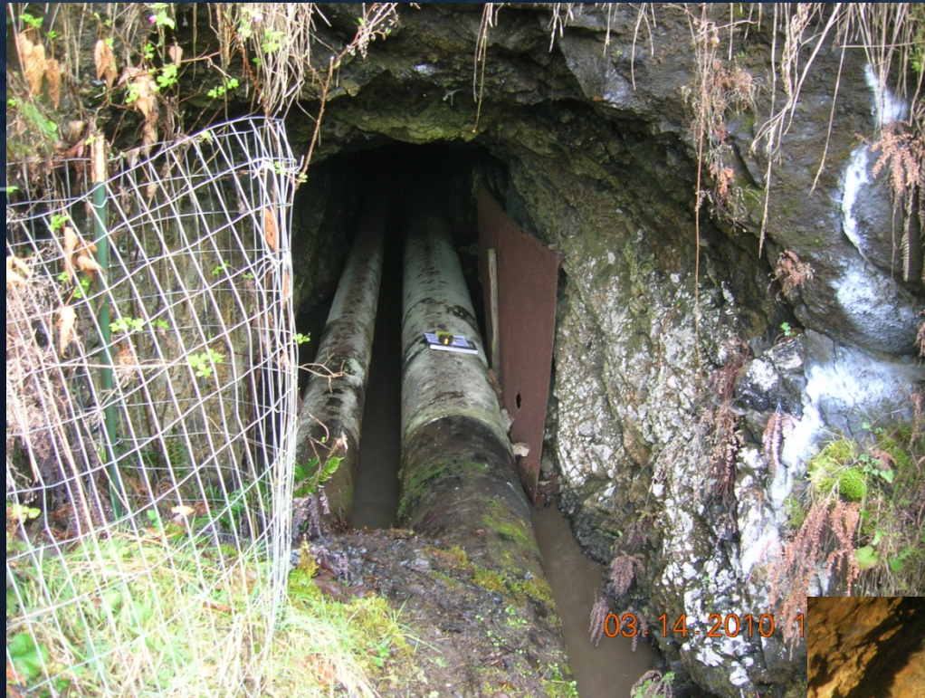
Tunnel Entrance with 24" Outlet Pipe and 16" Drain/Overflow Pipe
