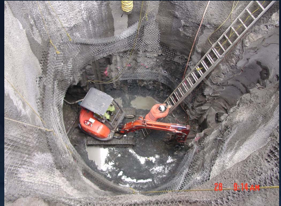
Operating at the bottom of the excavated shaft
