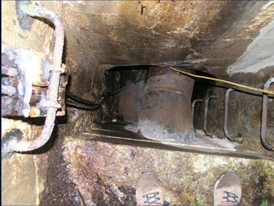
Overflow, Wet Shaft
