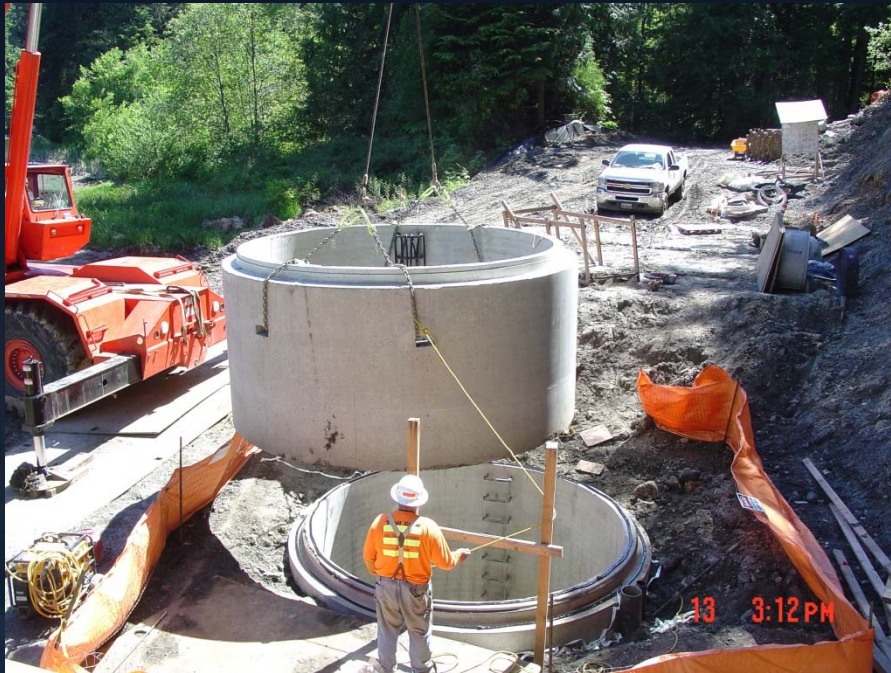
Installing 12-foot diameter precast segments
