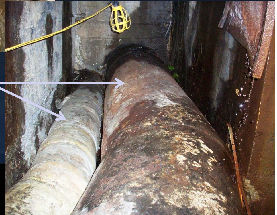
Outlet pipe and Overflow/drain pipe at bulk head inside tunnel
