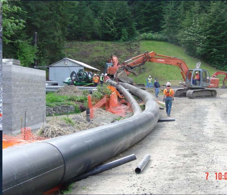
28" Outlet Pipe and 16" Overflow/drain pipe (HDPE)
