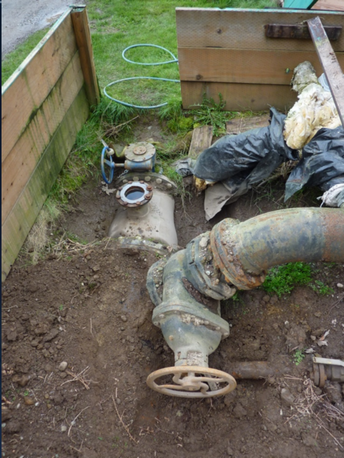
20" Isolation Valve for Current Flow Control (Manual , Cavitating )
