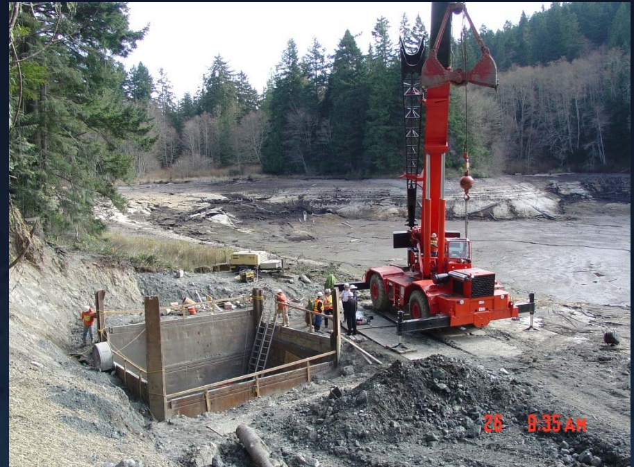
Excavation in soil w/ slide rail shoring system at new Control Shaft site
