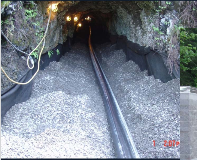
Drain Pipe at the bottom of Dry Tunnel
