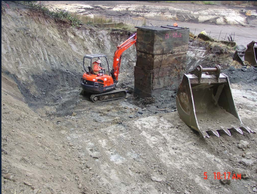
Excavating around Existing Control Shaft
