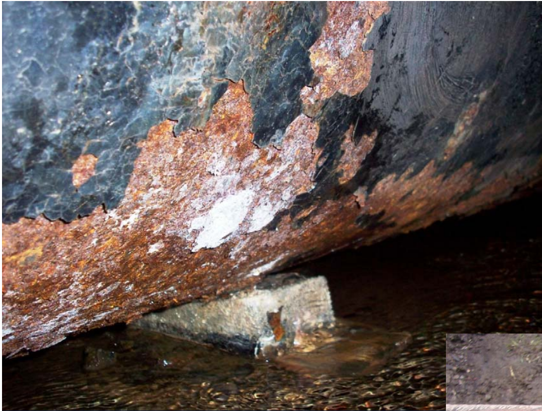
Corrosion of Drain Pipe
