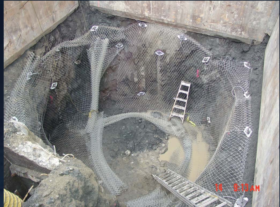
Rock dowels and netting to stabilize exposed rock inside shaft
