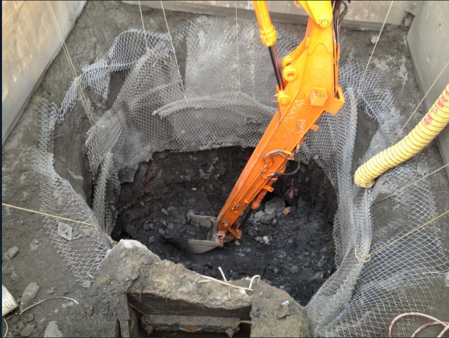
Excavation of rock from the surface
