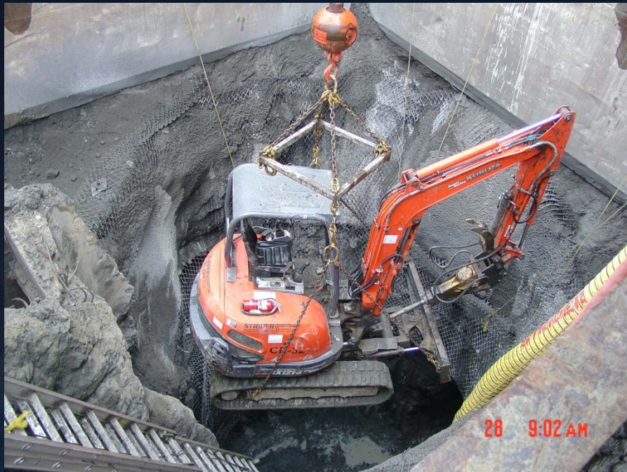
Lowering equipment inside the shaft
