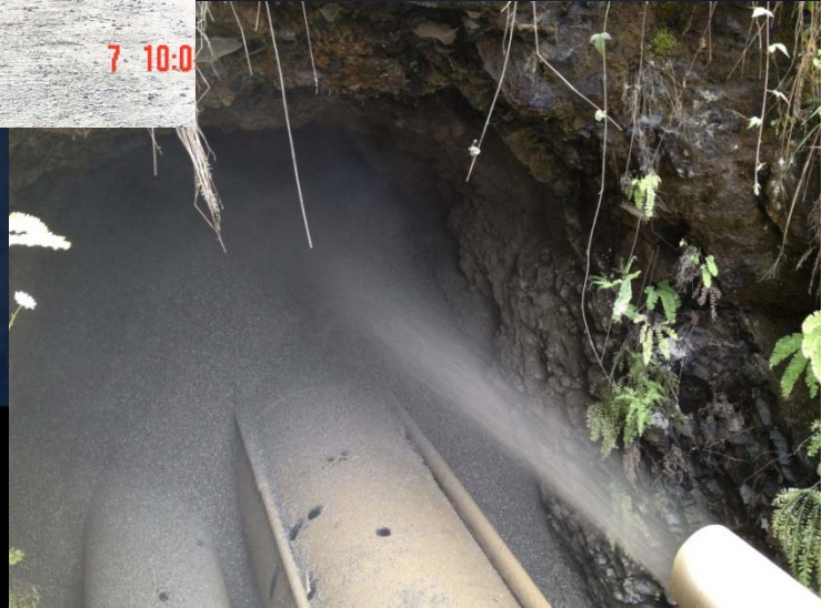
Blowing backfill inside dry tunnel
