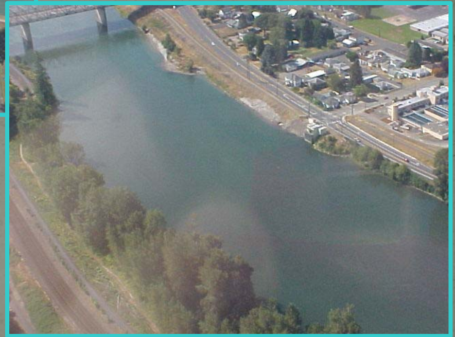
Longview Regional Water Treatment Plant and Intake September, 2005
