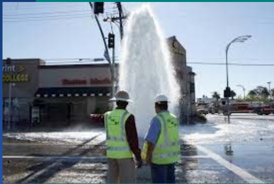
Water Main Breaks
