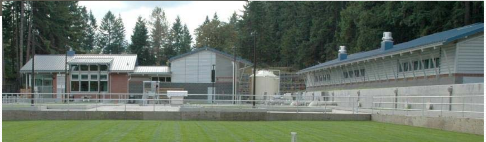
Martin Way Satellite Reclaimed Water Plant
