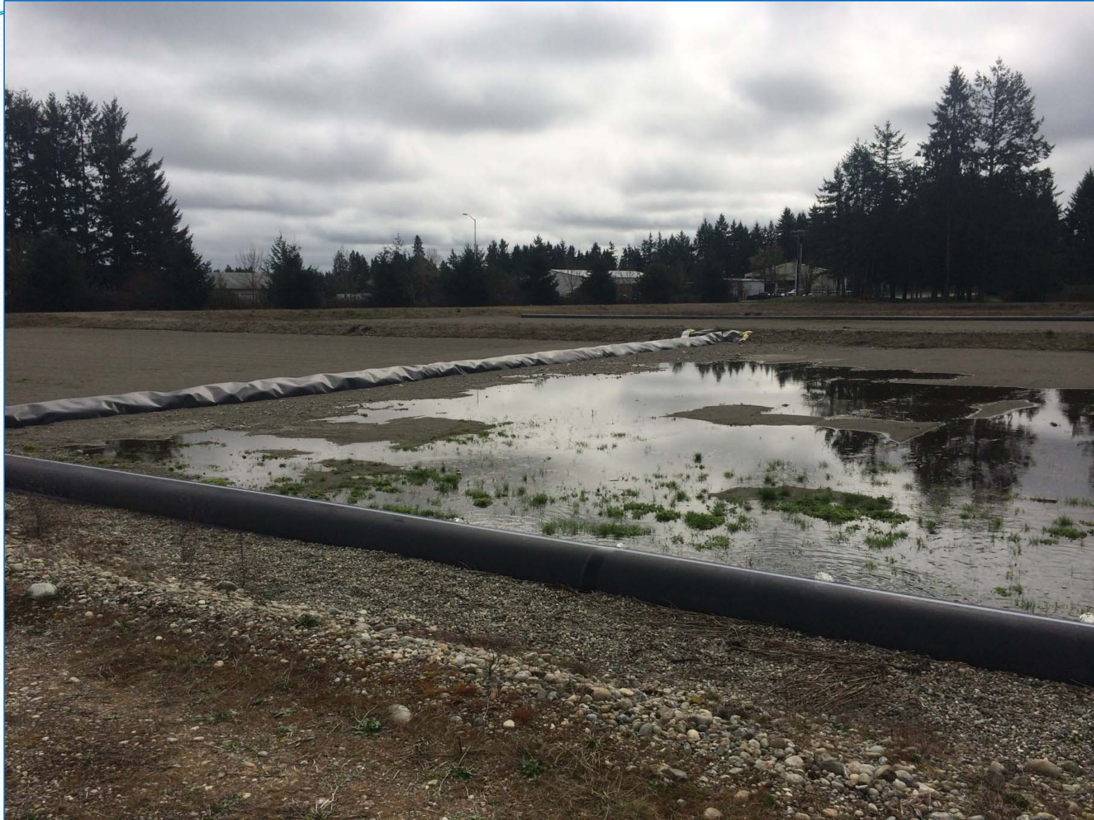
Basin 4 (looking SE, divider berm on left)
