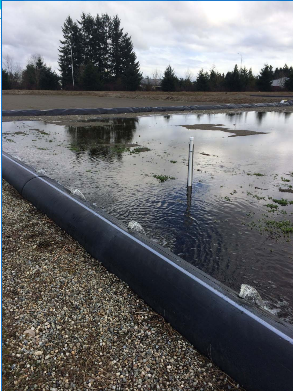
Basin 4 (looking SE, stilling well in foreground)
