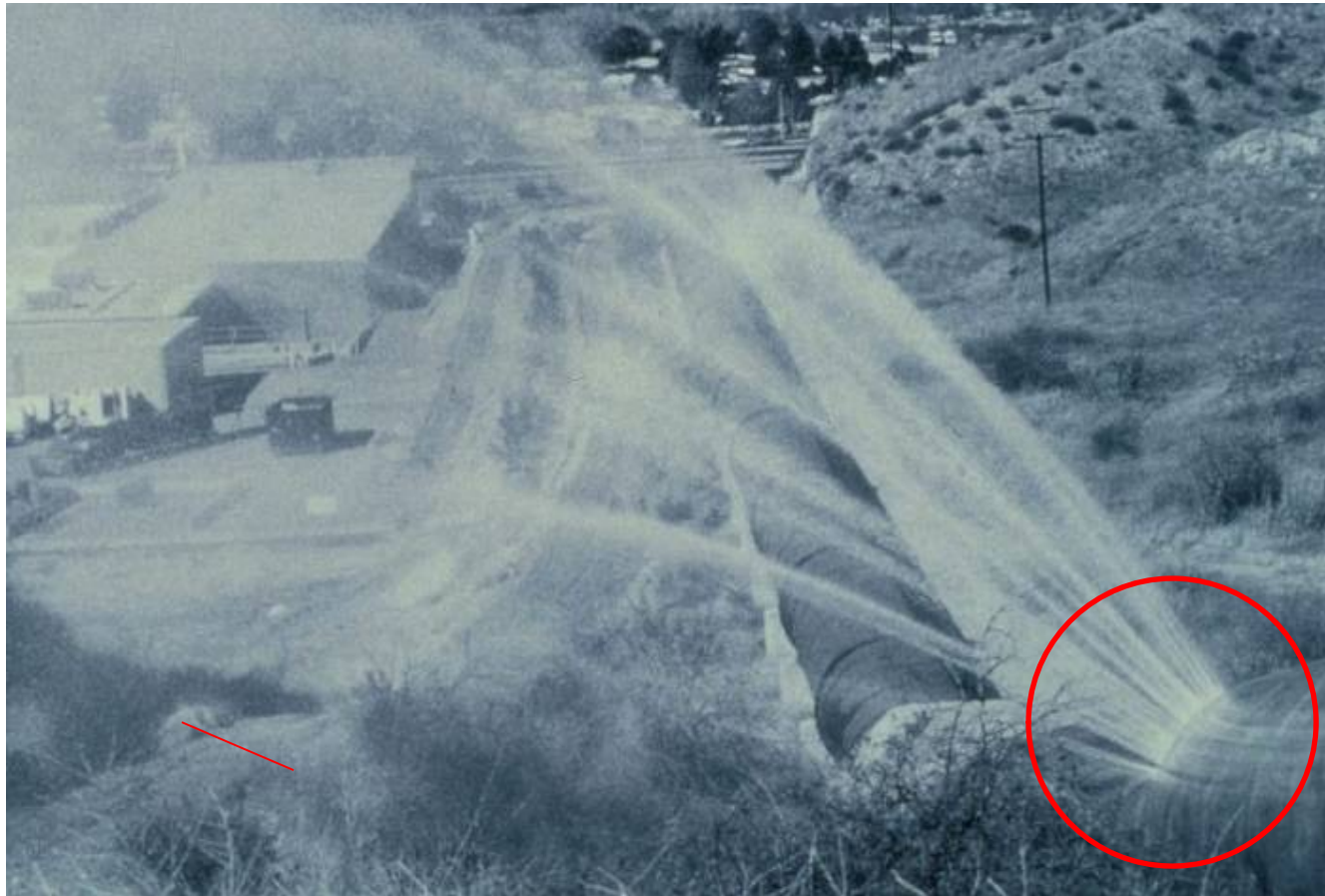
Rupture in 120-inch Soledad Siphon (1994 Northridge Earthquake)
