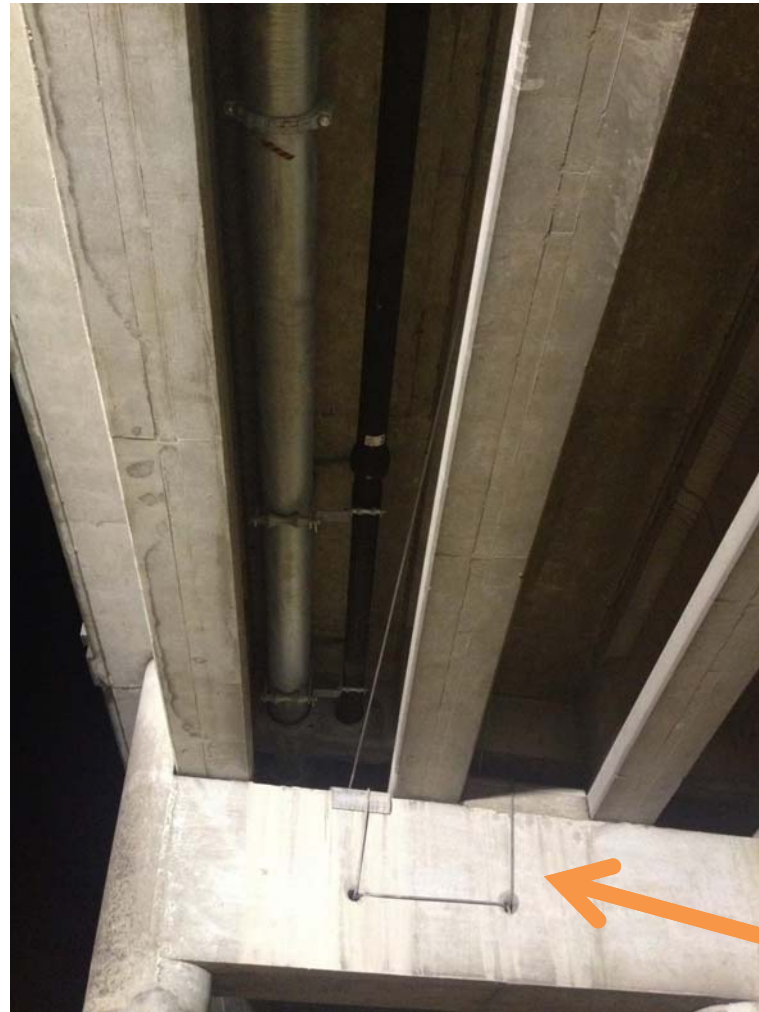
Bridge retrofit seismic cables
