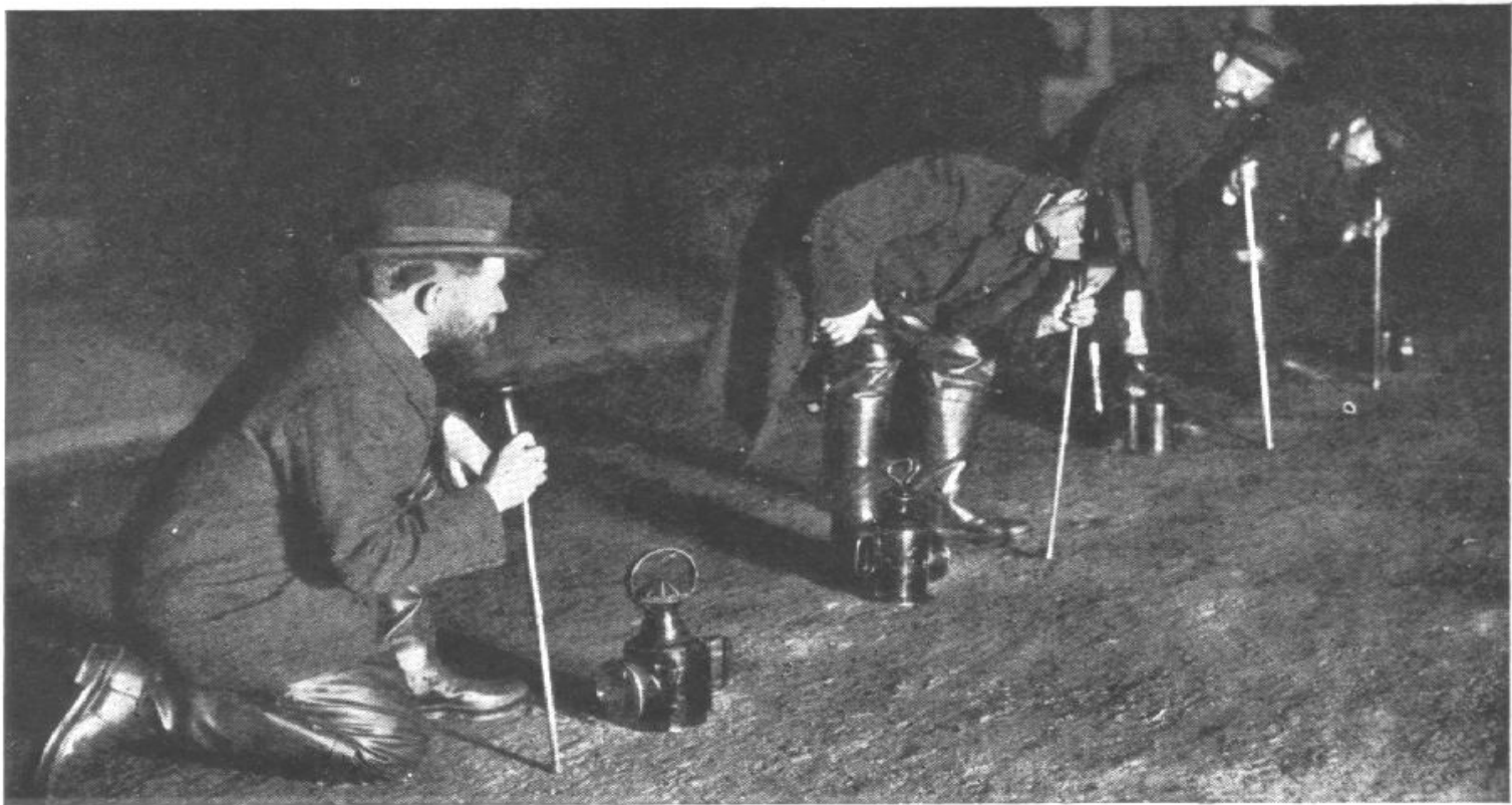
LISTENING WITH STETHOSCOPES AND AQUAPHONES ALONG A MAIN SUPPLY PIPE DURING A NIGHT INSPECTION.
