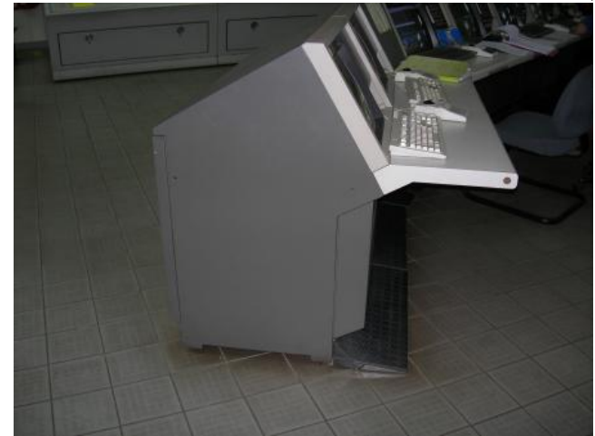
DCS Pre-Windows '80s (Bailey)
