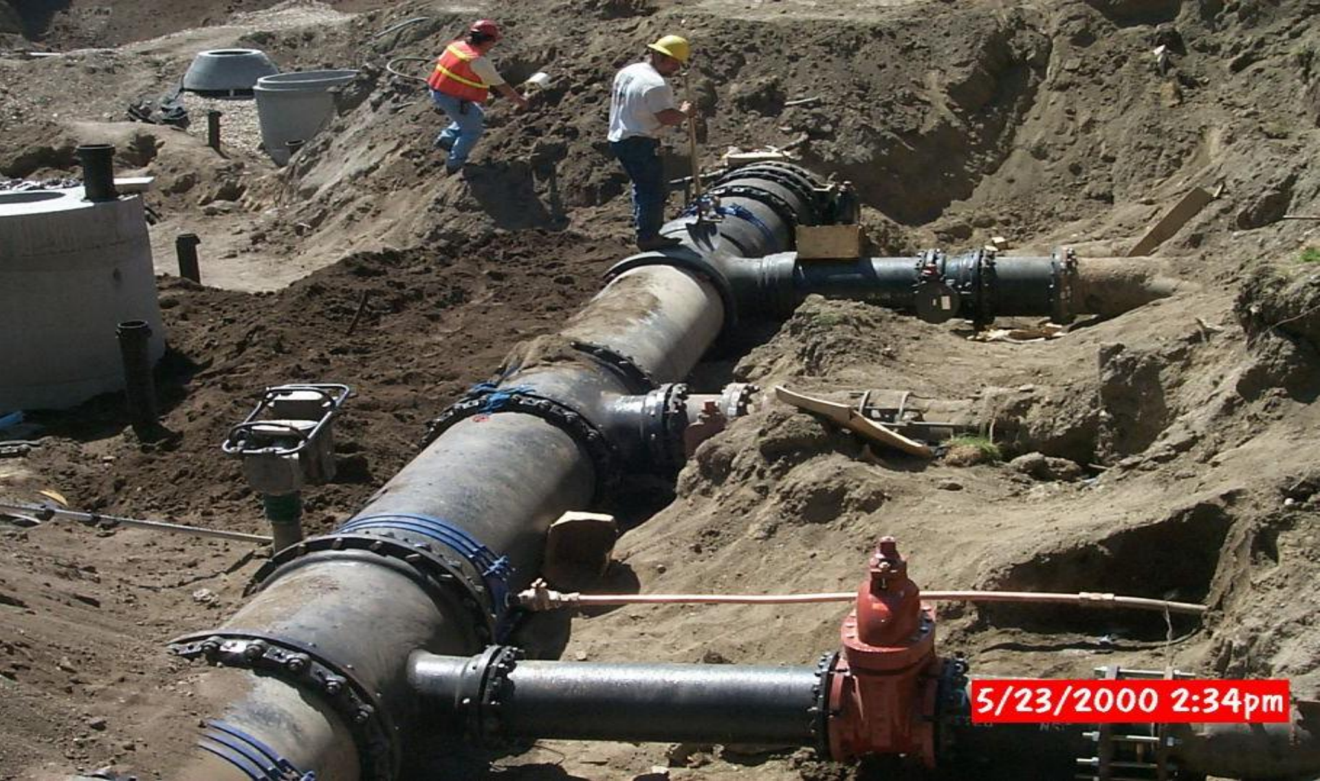
Construction of the discharge header
