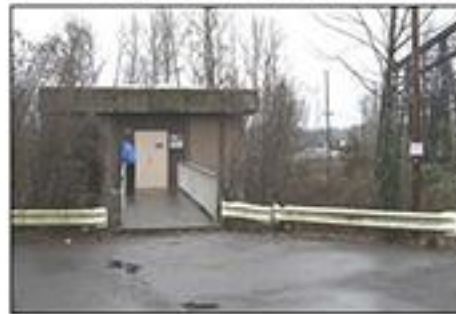
Existing river intake pump station:
