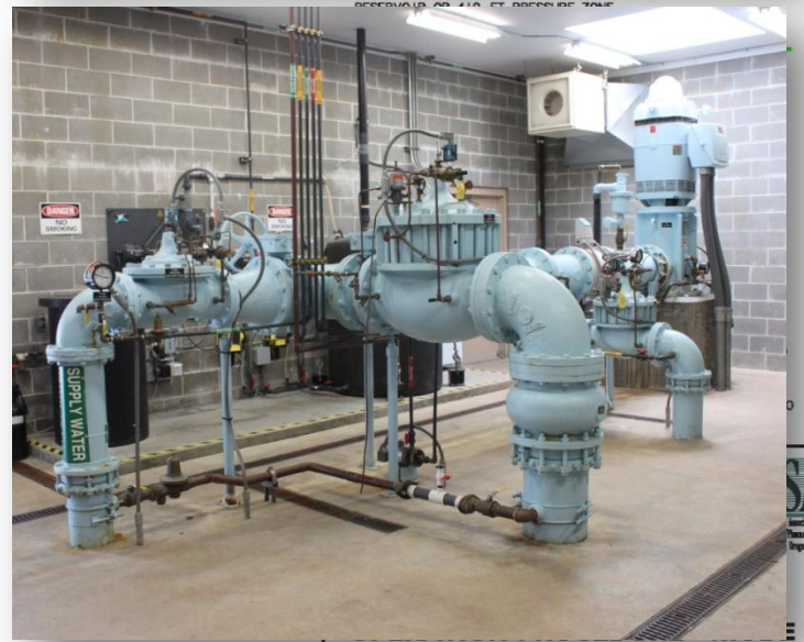
MODE 1B: ASR-2 DISCHARGE PIPING TO SUPPLY 10 MG RESERVOIR AT 410 FT PRESSURE
