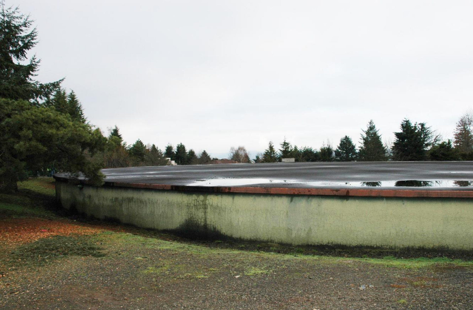
ROOF CRACKING AND SAGGING ALLOWED RAIN WATER TO ENTER RESERVOIR
