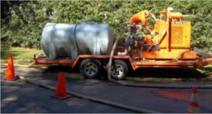
Pressurization tank used to force pig from launcher into water main
