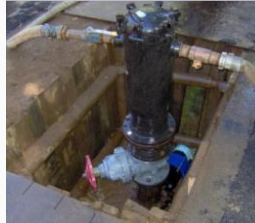
Pig launcher installed in street, on 'T' fitting
