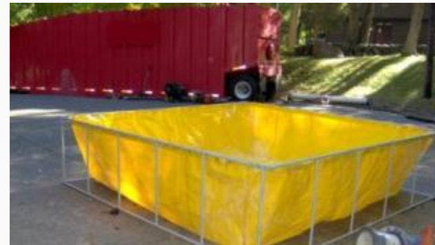
Temporary catch basin and disposal truck
