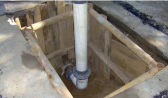
Recovery point at end of main (modified blow off)
