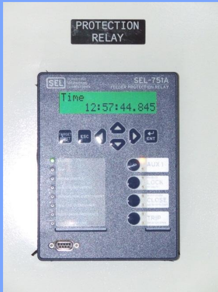
Utility Required Relay - SEL-751A
