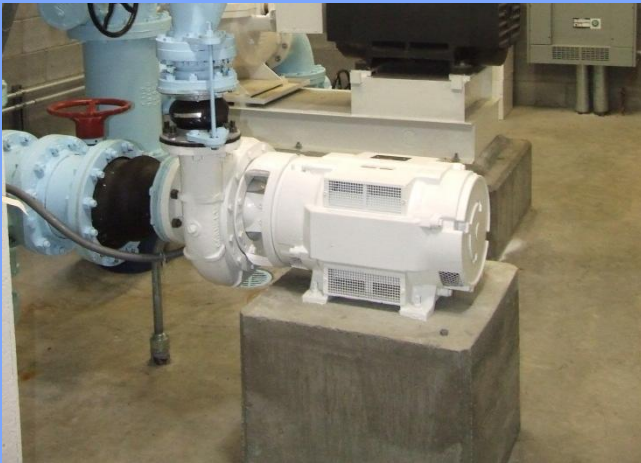
Well 5 – 50 kW Micro-turbine
