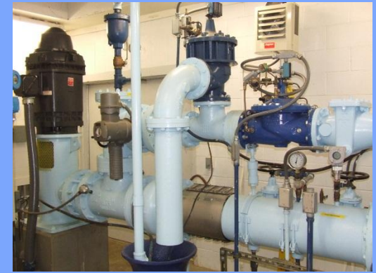
100 HP Motor, Valves, Piping, Etc.
