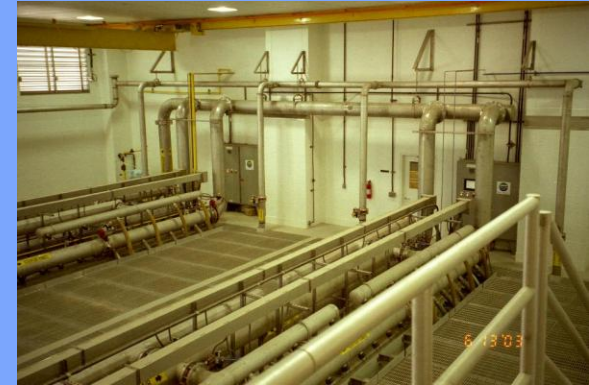
2003: WTP Membrane Room
