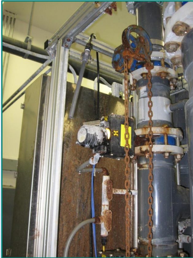
Rack Corrosion
