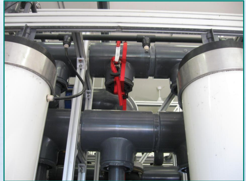
PVC Header Damage
