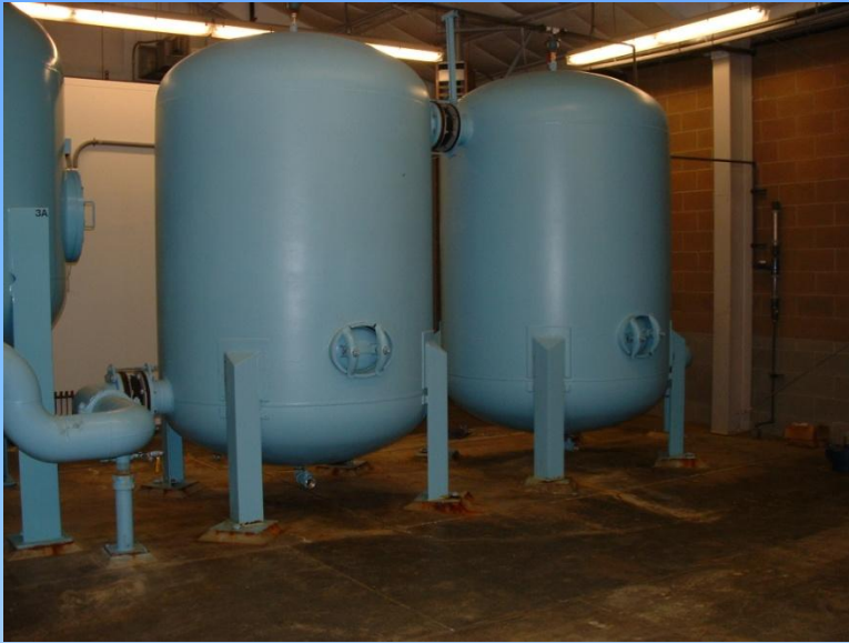
Ozone Contact Tanks
