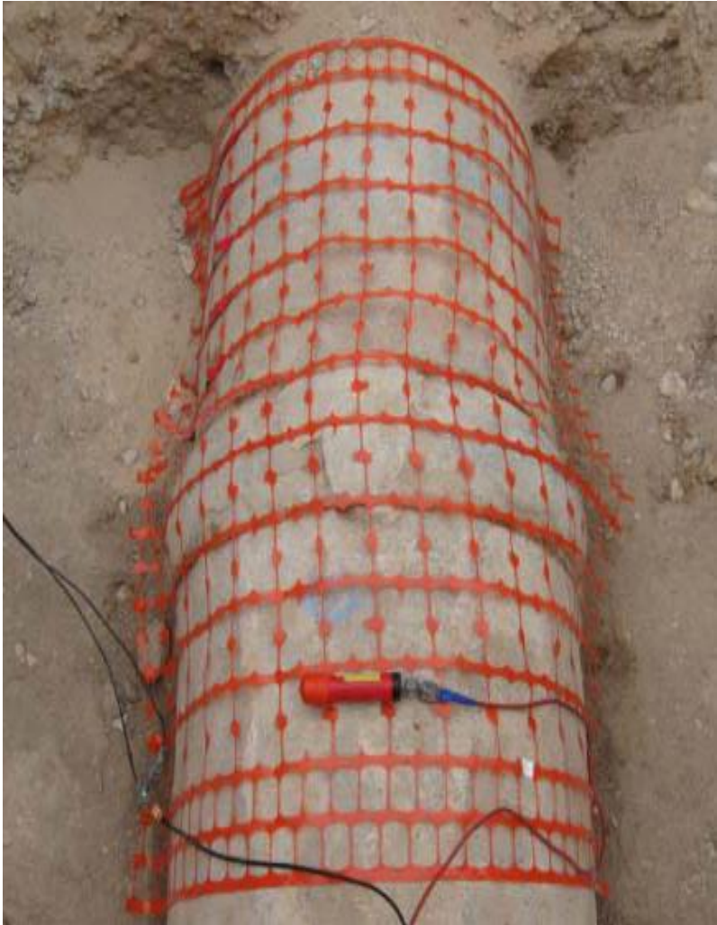
External Corrosion Direct Assessment
