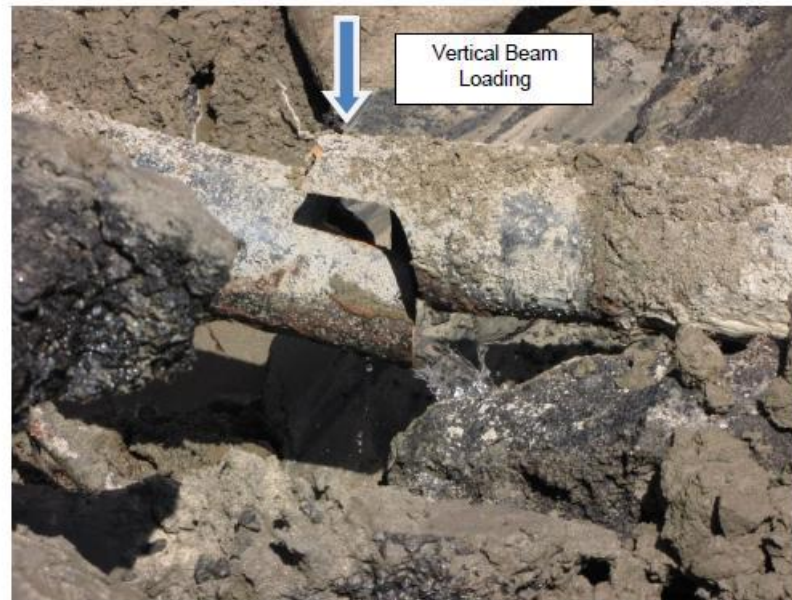
Figure 3-3. "Circular Break" (Circumferential Crack Propagation) due to beam loading at 12212 Hartsook Street (Figure 2-2)
