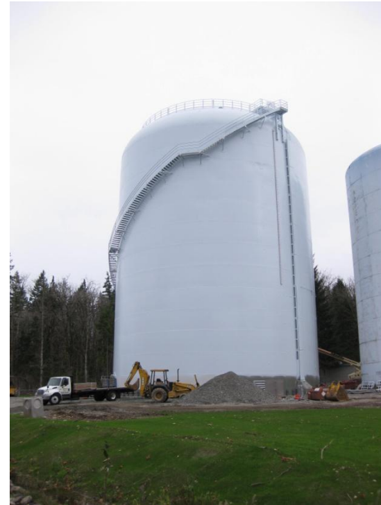
Tank Painted – Back in Service
