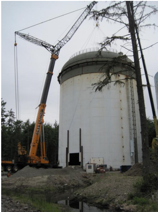
Roof in Place – Ready to Weld
