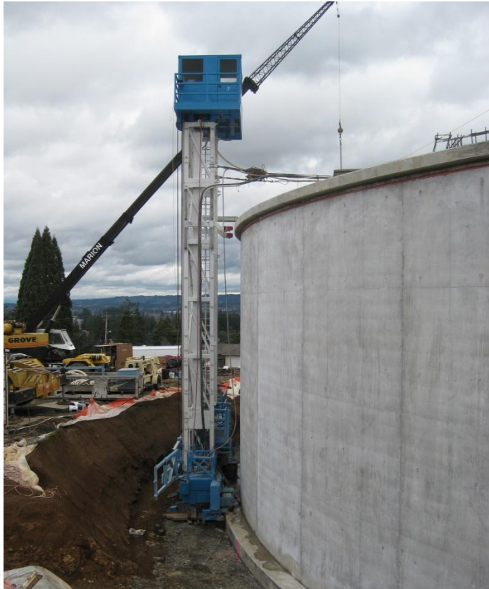
Circumferential Prestressing Machine (Wrapping Machine) Preparing to Wrap Strand
