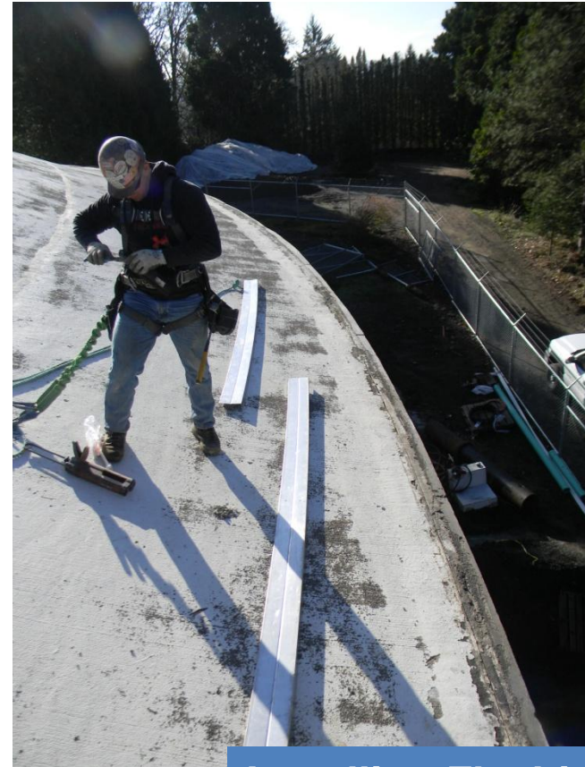
Installing Flashing
