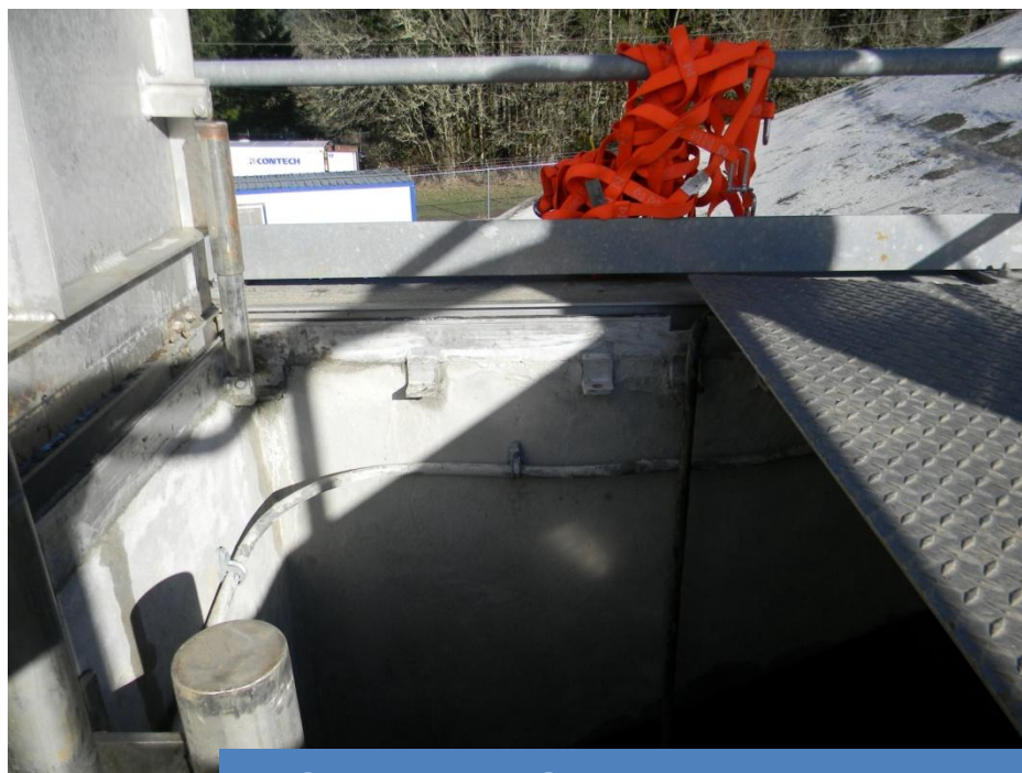
Concrete Surface Repair and Coating of Inside Access Hatch
