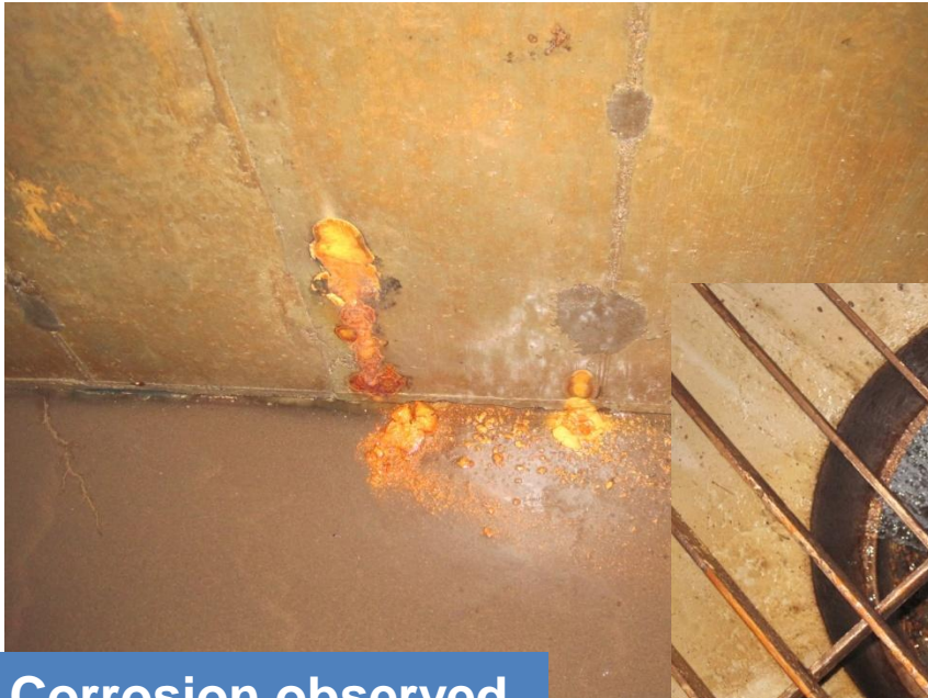
Corrosion observed Determined not to be rebar
