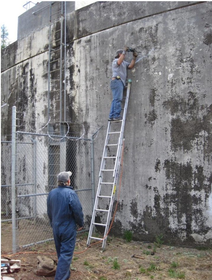
Exposing wire wrap for inspection
