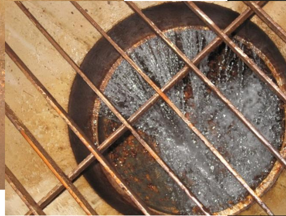
Inspect ladders, overflow, drain and other appurtenances
