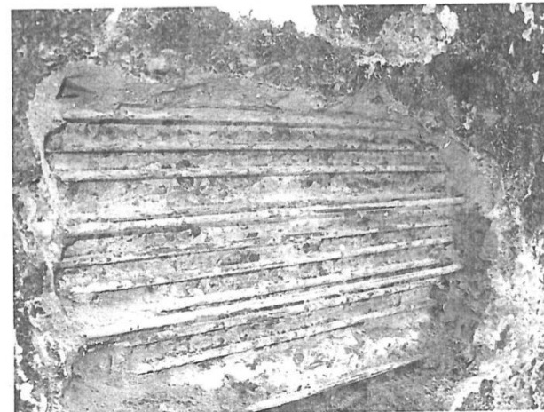
Photo No. 10. Bellhole No. 7.
