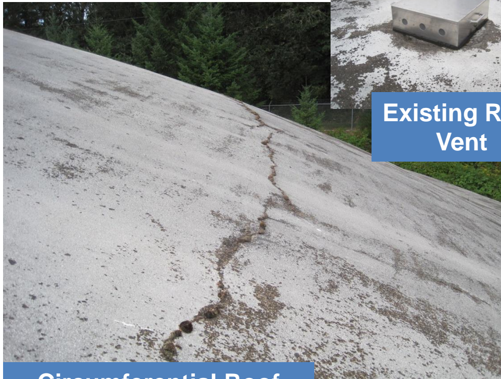
Circumferential Roof Cracks Observed
