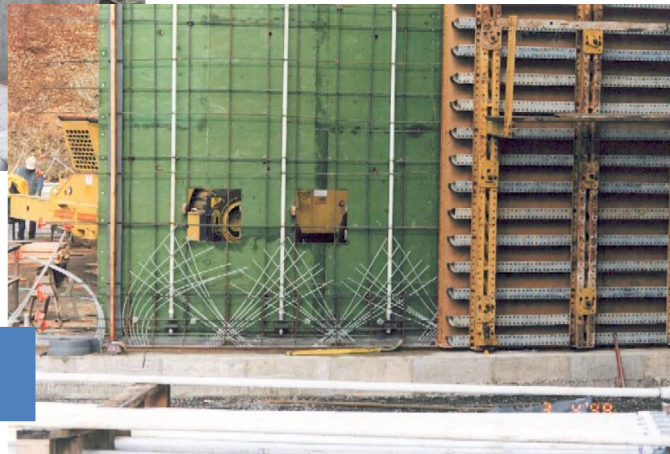
Forming for Core Wall: Note Seismic Cables Cast in Footing
