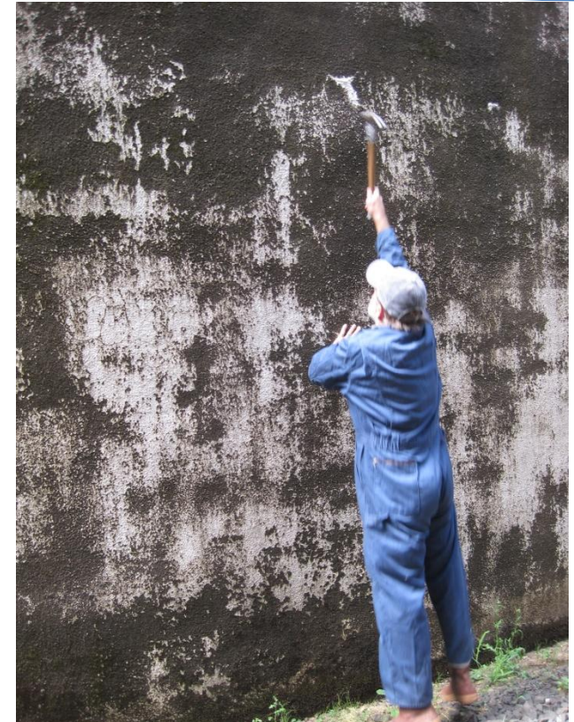
Sounding shotcrete to locate voids that identify delaminating areas
