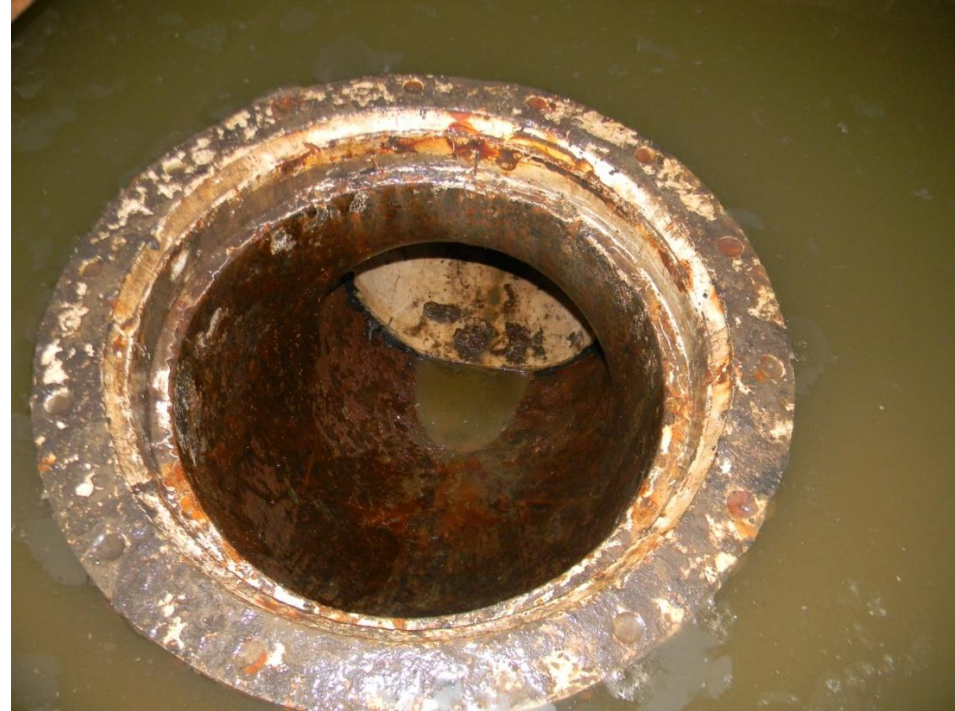
CIPP Cured, Trimmed and Sealed at Reservoir Floor Sump
