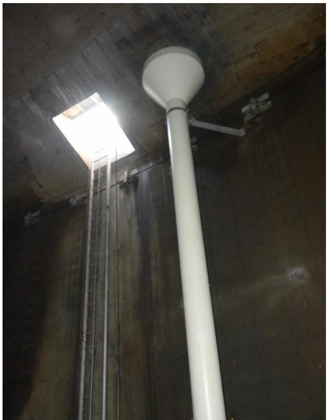
New SS Ladder and Painted Overflow Piping
