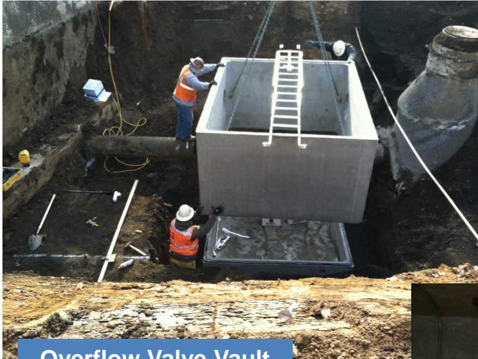
Overflow Valve Vault
