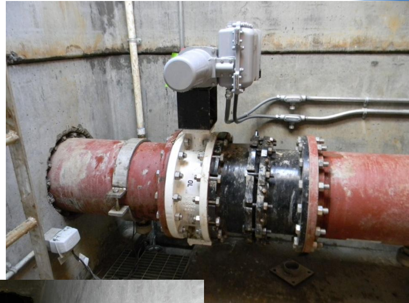
Seismic Controlled 16-inch BFV with 120 VAC Motorized Actuator and UPS
