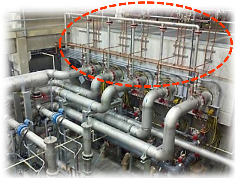
Enaville– Air Removal System ( Pressure Venturi Ejectors )
