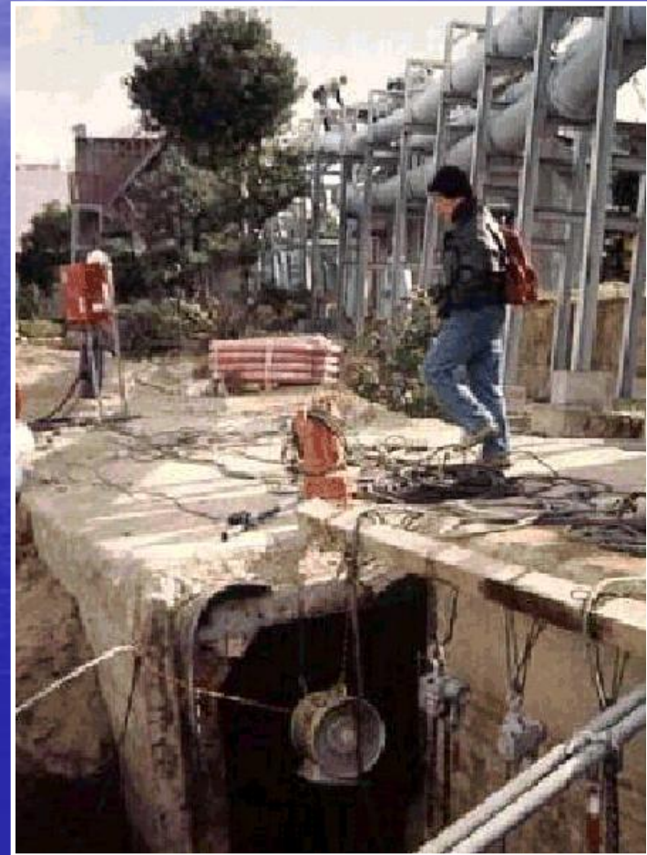
Higashinada WWTP, KObe Japan, 1995. 2 meters lateral and 1 meter vertical movement
