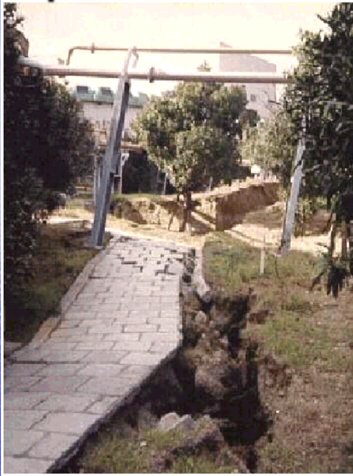
Higashinada WWTP, KObe Japan, 1995. 2 meters lateral and 1 meter vertical movement
