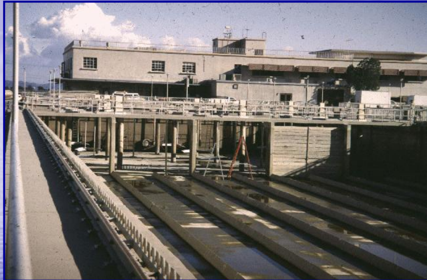
Jensen WTP 1994 Sedimentation Tank Damage
