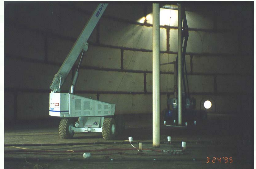
Propane-powered manlift in a large tank
