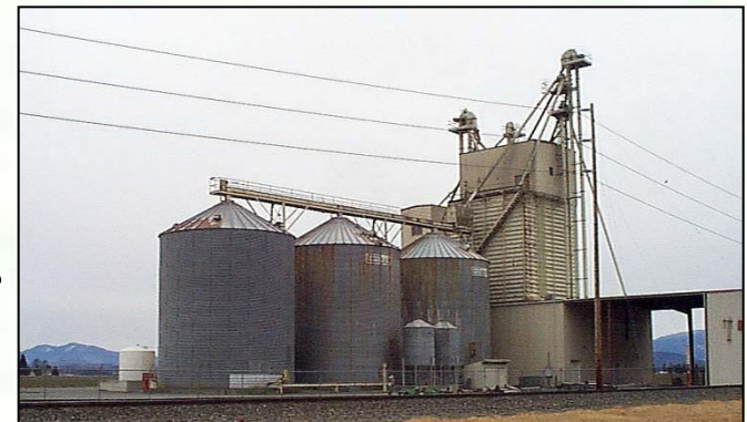
Grain storage bins
