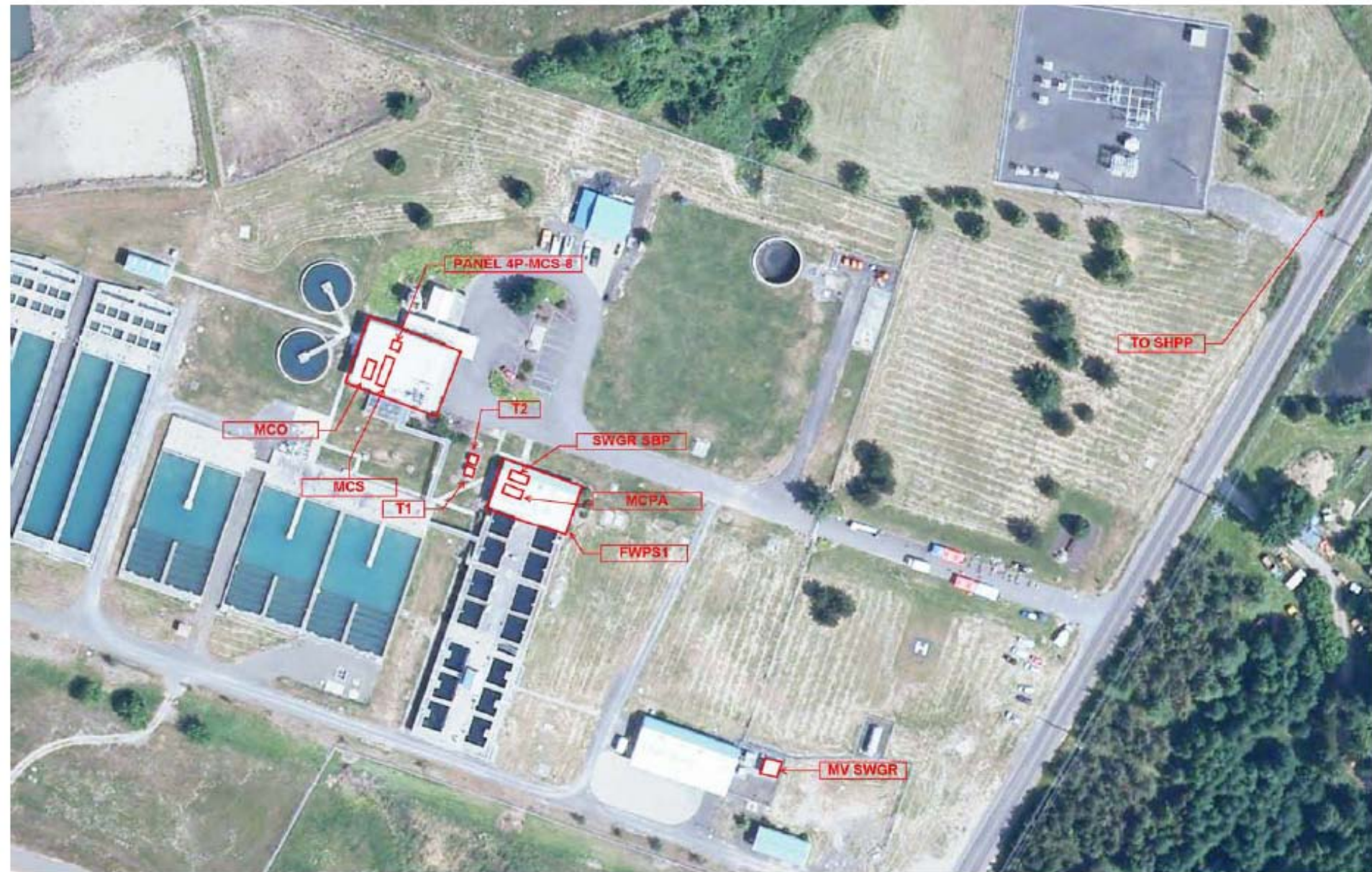
Figure 1: Aerial photo of the Water Treatment Plant
