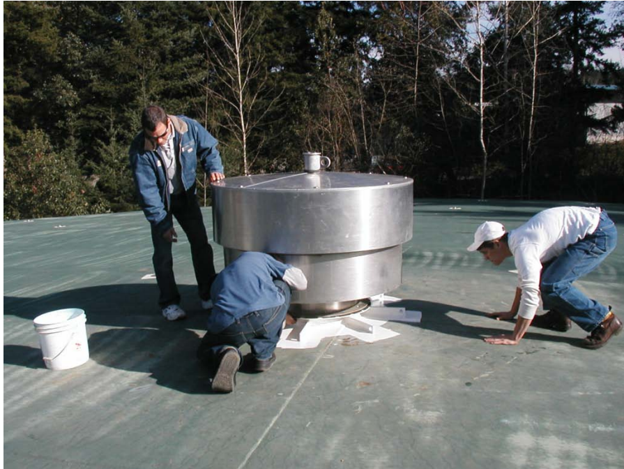
New Vent with modified Fall Protection
