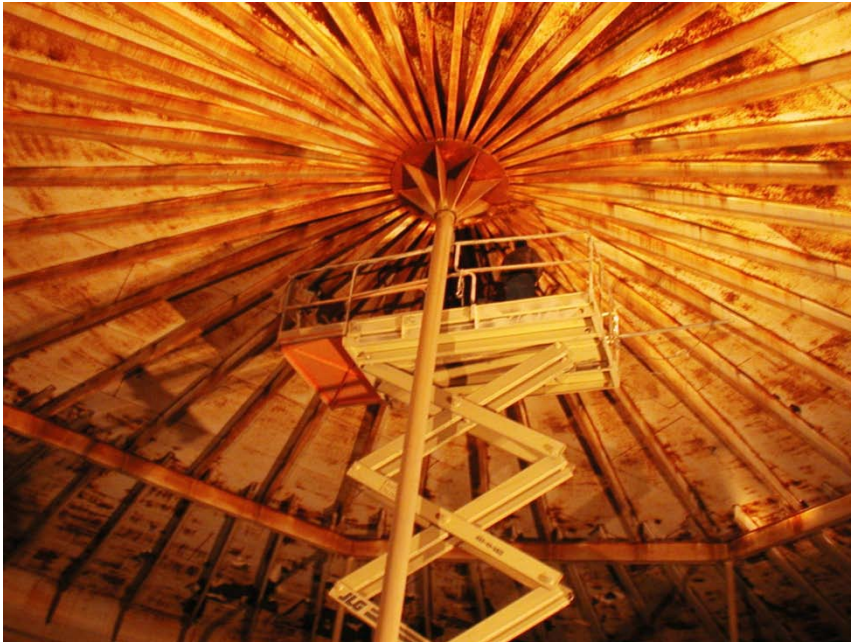
Rafter Beam / Roof Plates -- Before
