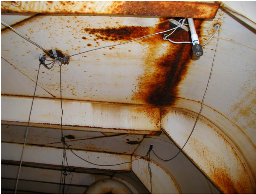
Rafter Beam / Roof Plates -- Before
