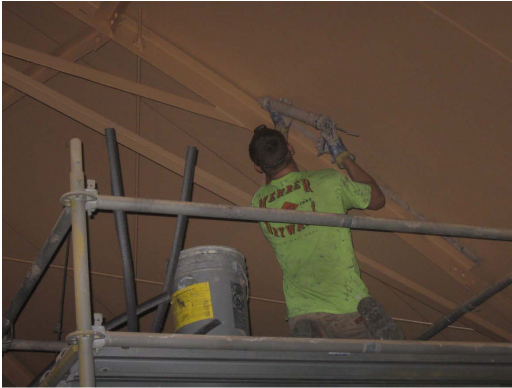
Caulking between Truss and Roof Plates
