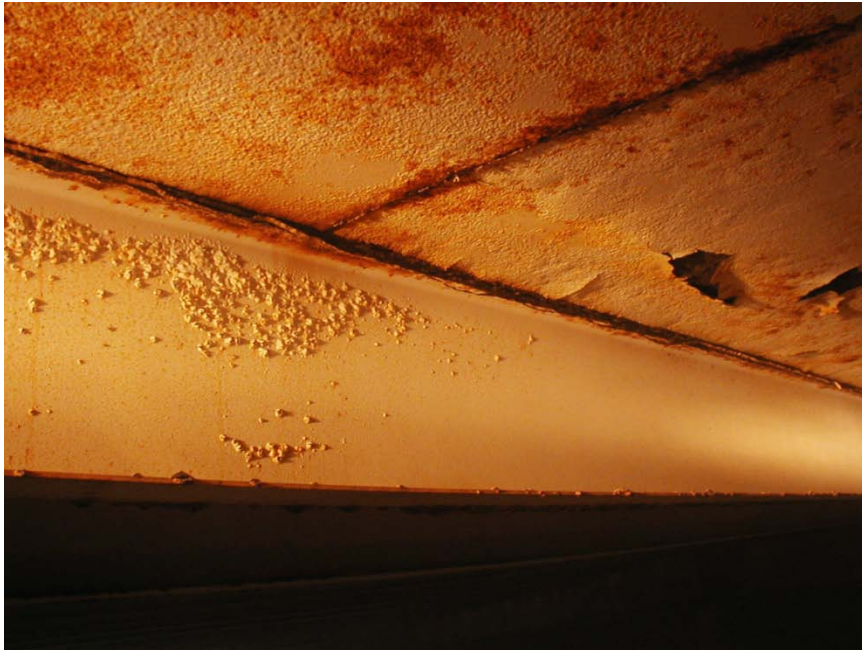
Rafter Beam / Roof Plates -- Before
