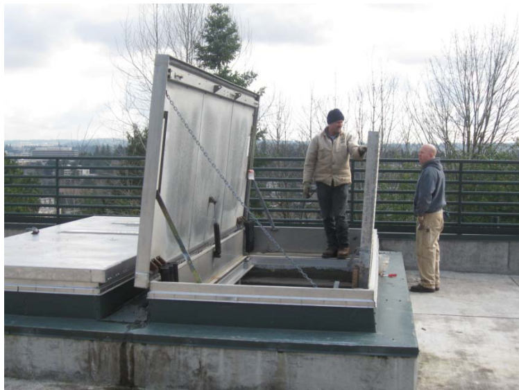
Hatch Components – Corrosion after 7 years
