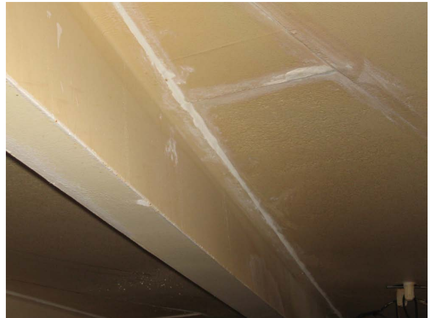
Rafter Beam / Roof Plates w/ Caulking after 7 Years
