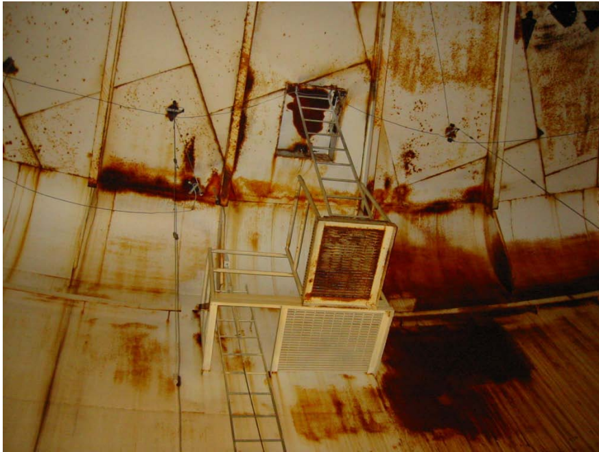
Ladder / Landing -- Before
