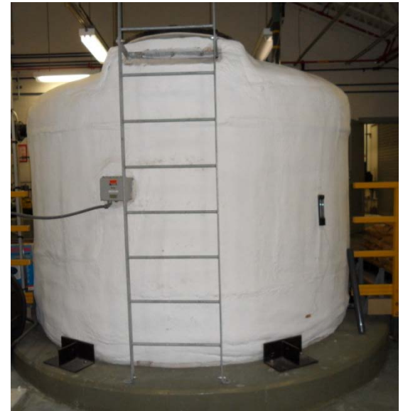
Bulk storage of 50% caustic soda at District treatment site
