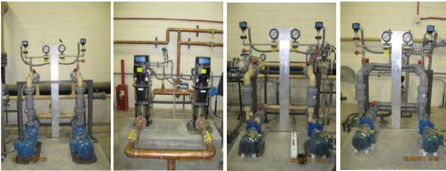
Zone 4 Groundwater Treatment Plant Glendale Arizona
