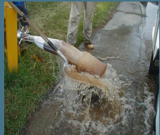
Flushed Deposits Captured in Hydrant Nets
