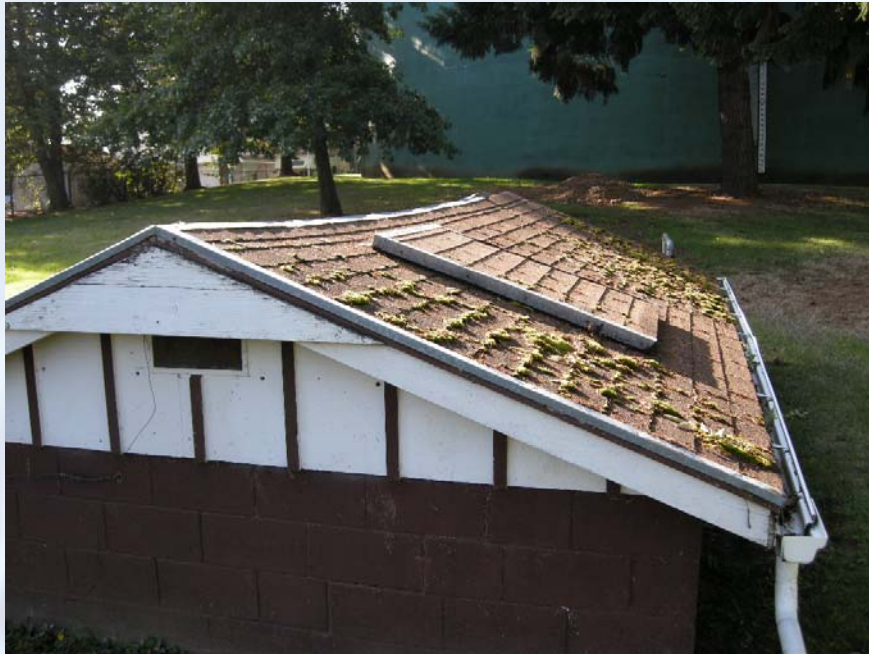
Original Pump Station
