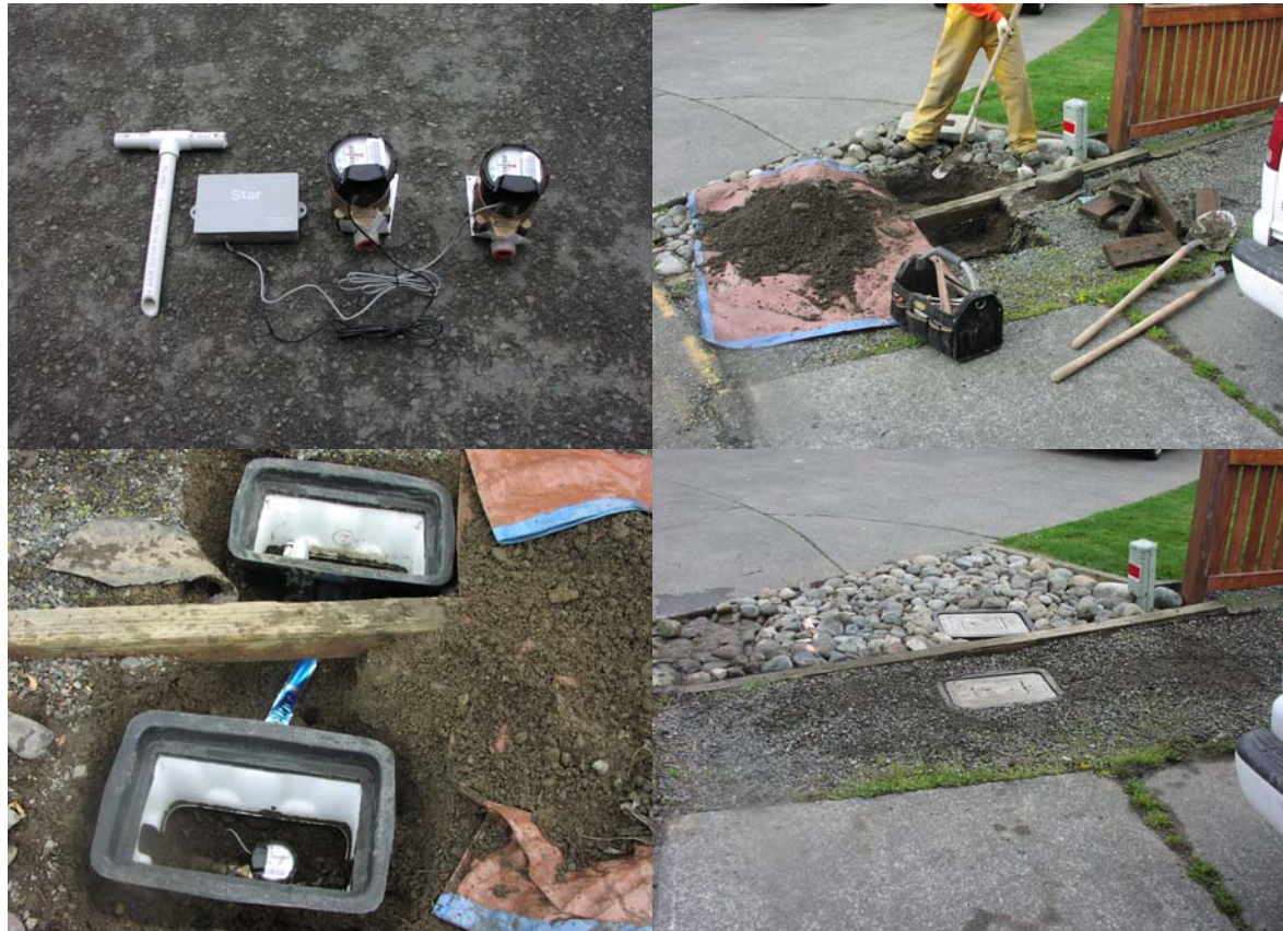
Meter Transmitter Unit (Dual Meter) + Meters and Registers
