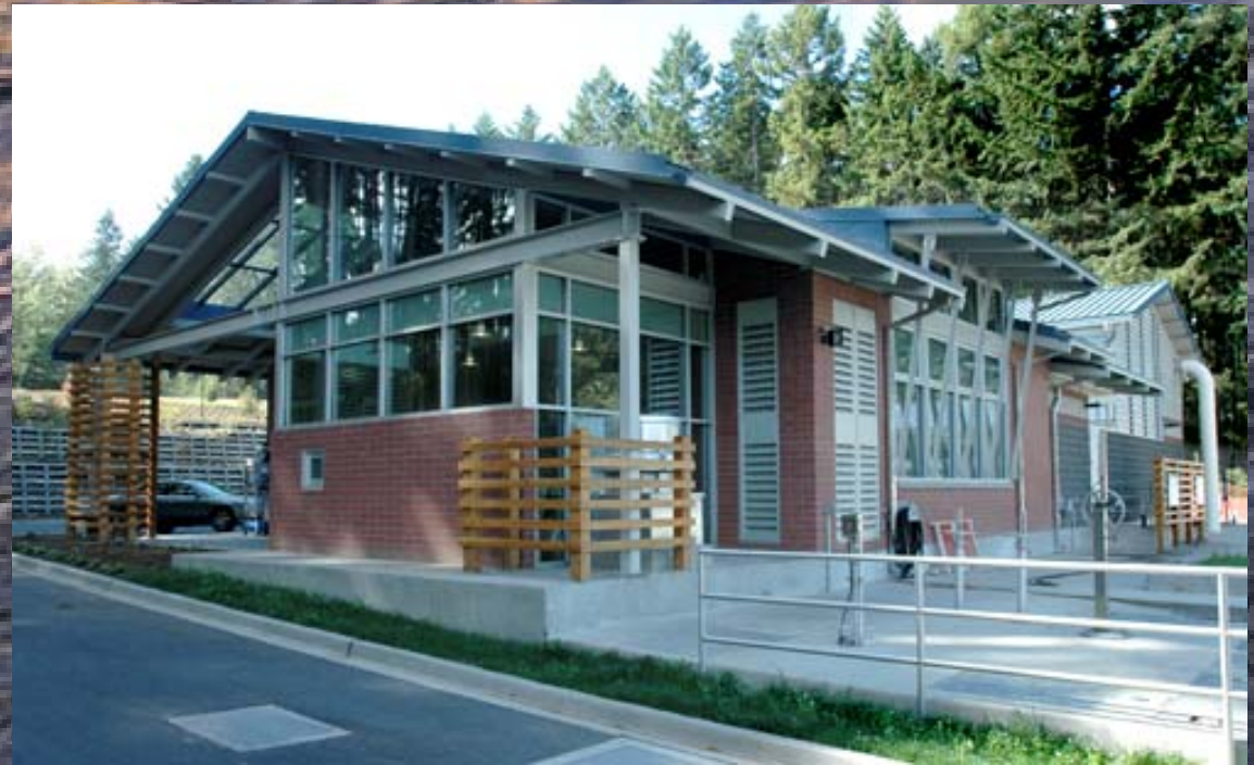
Operations & Headworks Building
