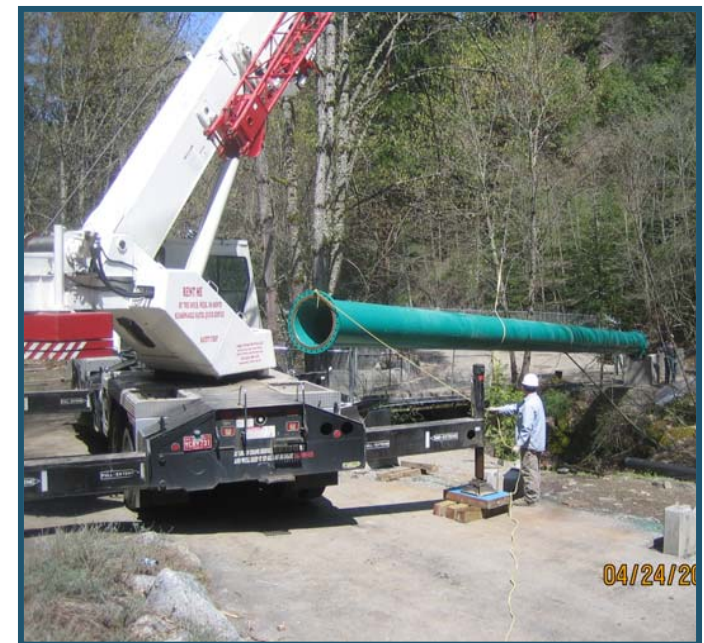
30-Inch Wash Water Pipe Installation Above River
