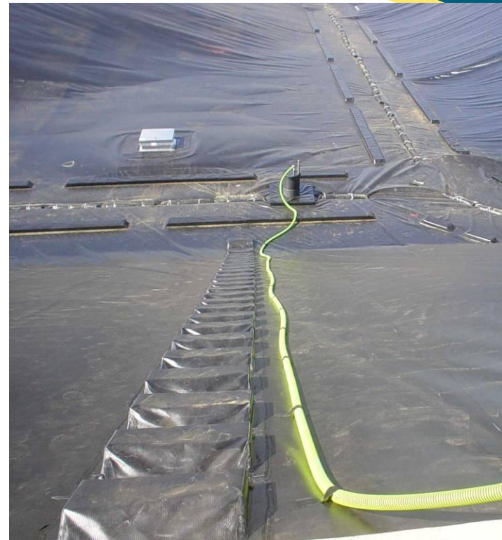
Walkway to Hatch/Sump Pump
