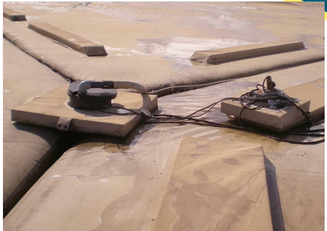
Sump Pump Assembly
