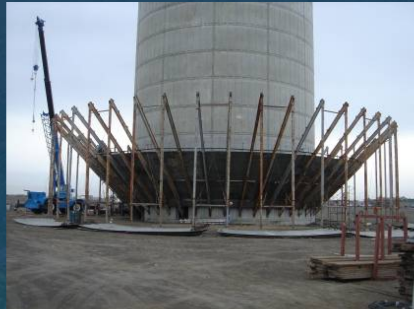
Rig and Beginning Welding the Cone Portion of the Reservoir
