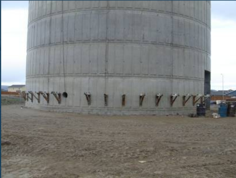
Set the Ring Beam Supports
