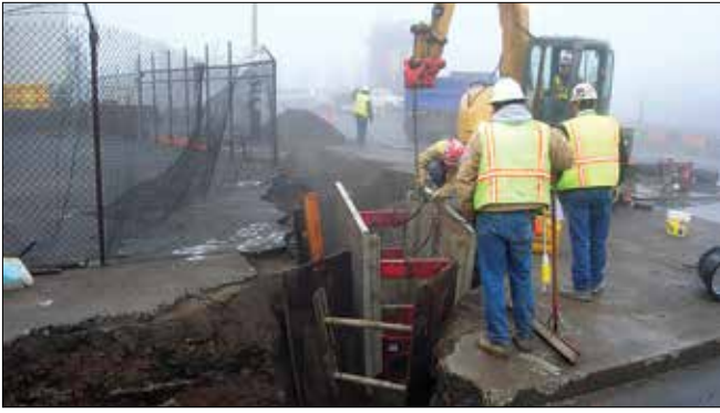
Figure 2: Shoring can prove to be challenging in streets that are congested with other utilities. Photo Credit: Portland Water Bureau
