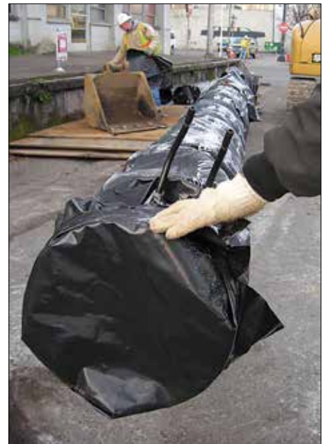
Figure 6: Polyethylene encasement provides additional protection from corrosion. Photo Credit: Portland Water Bureau
