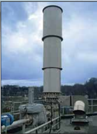
Enclosed Waste Gas Burners
