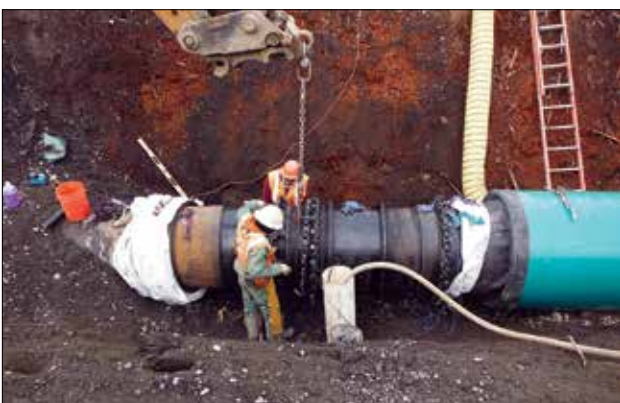
Figure 7: Several large-diameter transmission mains were replaced and encased in steel casings. Photo Credit: Portland Water Bureau
