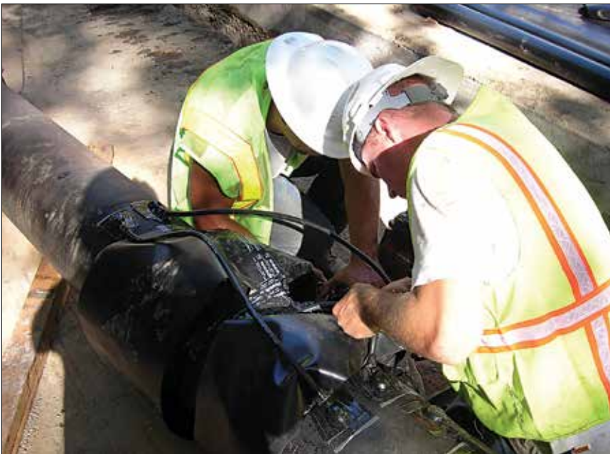
Figure 5: Bonding wires installed across each pipe joint creates a continuous electric circuit between corrosion test stations. Photo Credit: Portland Water Bureau
