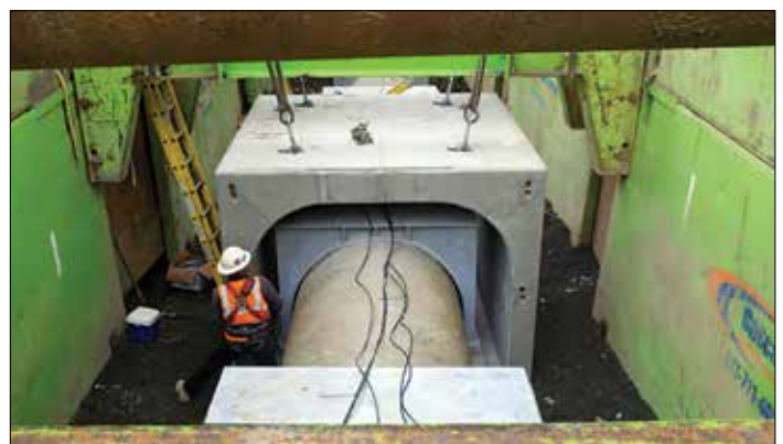
Figure 8: The Washington County Supply Line was protected in place with a pre-cast box culvert. Photo Credit: Portland Water Bureau
