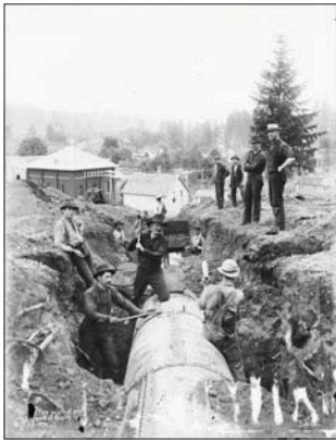
Seattle's Cedar River Pipeline 1 (1899)
