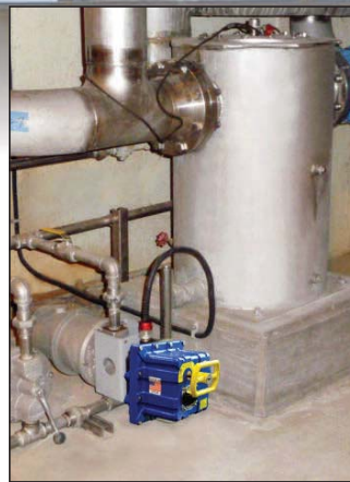
Sediment Trap with Electrically Actuated and Manual Drip Traps
