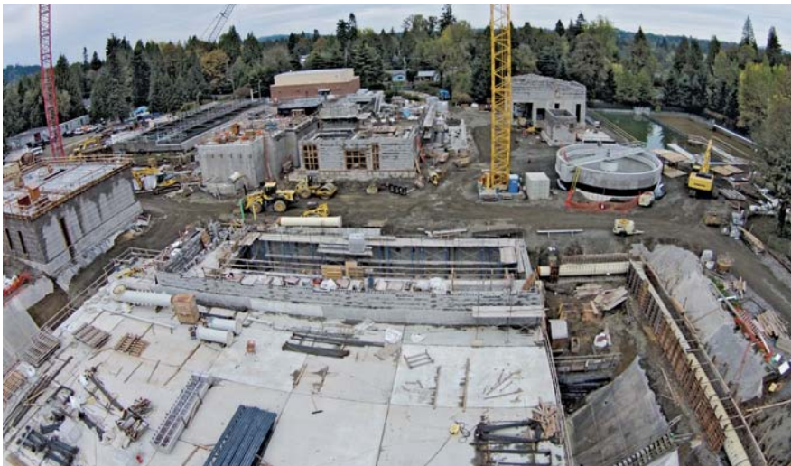
Foreground: 2 MG clearwell (to be buried) and finished water pump station. Left to right: electrical building, existing filters and sedimentation basins (to be removed), ballasted flocculation, chemical building. Right of yellow crane: solids handling, screw press and gravity thickener.
