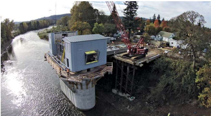
The new river intake pump station on the Clackamas River is held into bedrock with 14 ground anchors.
