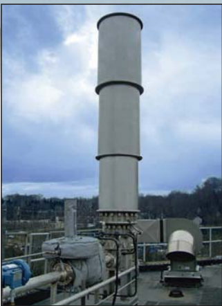
Enclosed Waste Gas Burners
