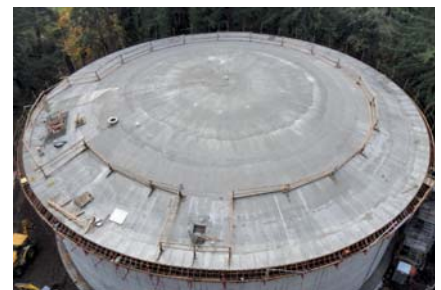
The new Waluga Reservoir 2 in Lake Oswego contains state of the art seismic design features.
